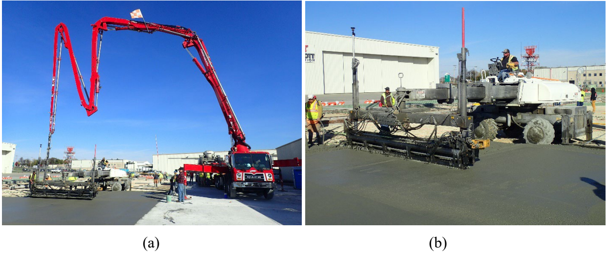
Figure 42. Laser Screenshot Applications via (a) Concrete Pump Truck and (b) Laser Screenshot
