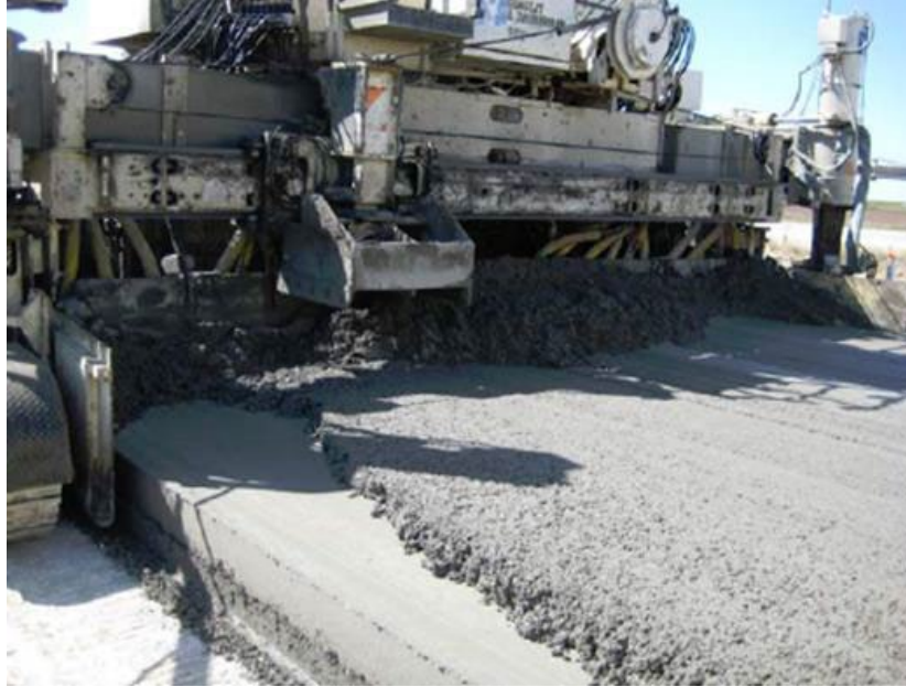
Figure 2. Two-lift Construction of Concrete Pavement in Progress (Hu et al., 2014)
