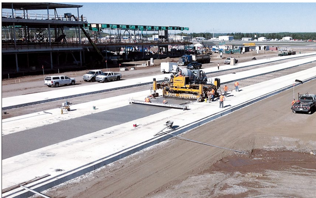
Figure 43. Slipform Paver (Photo Courtesy of Gomaco)
