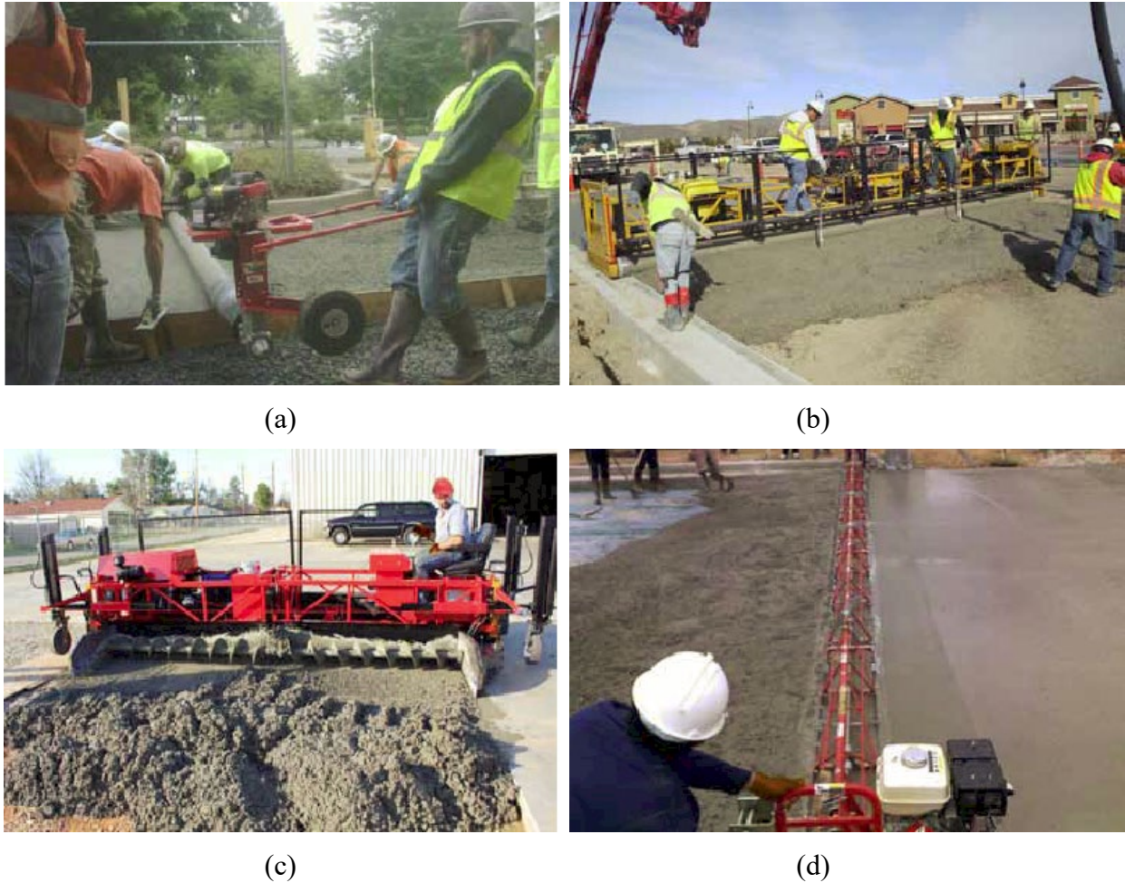
Figure 41. Placement Types: (a) Spinning Tube Screed, (b) Triple-roller Tube Paver, (c) Roller Screed, and (d) Vibratory Truss Screed (Harrington & Riley, 2012)
