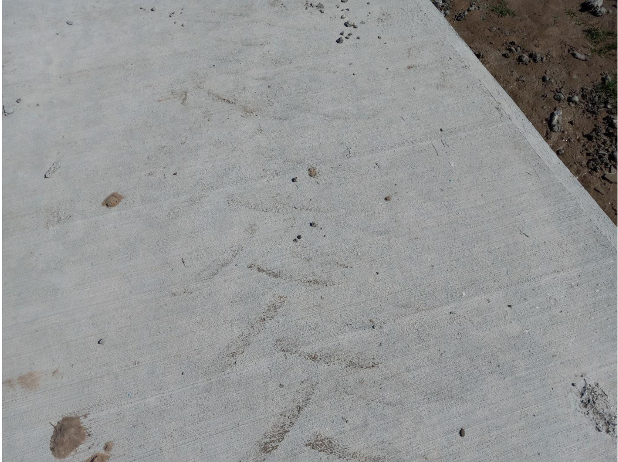
Figure 4-5 The finished surface of the concrete after the Pulp Cure naturally was removed.
