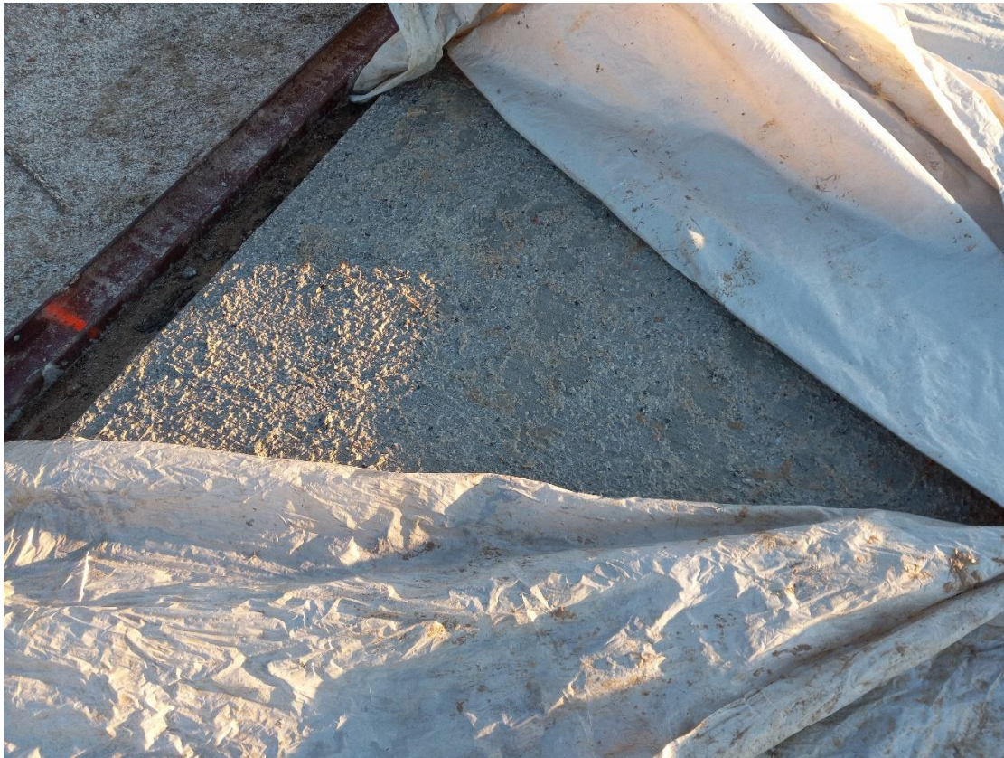
Figure 4-4 Pulp Cure applied at 1/4" thickness and then covered in plastic.
