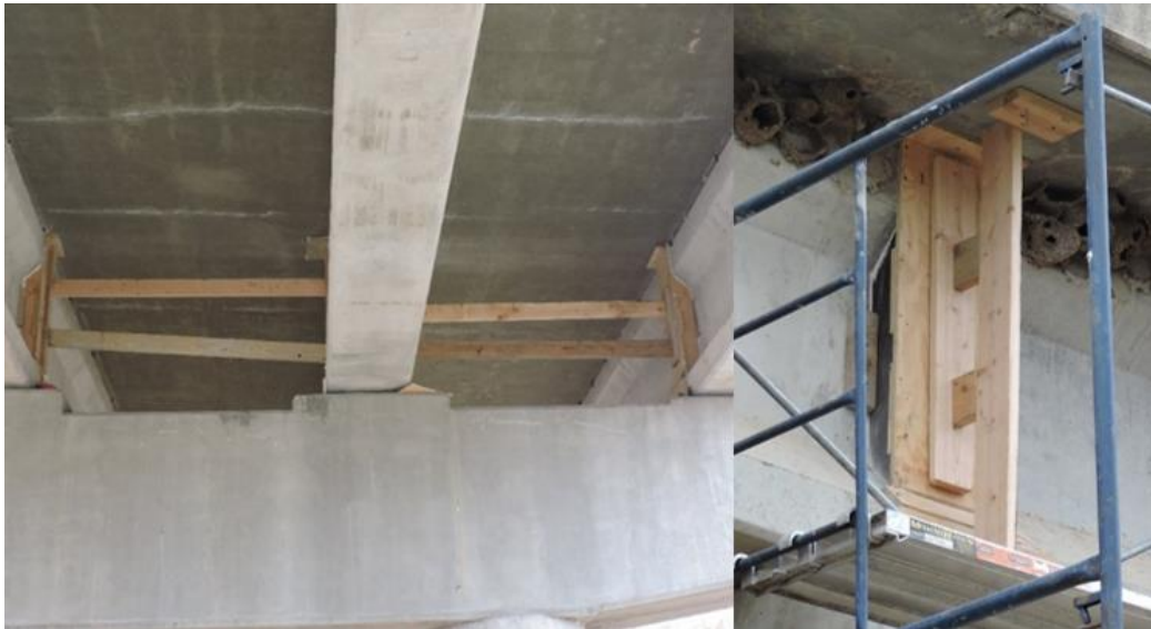
Figure 94. Final joint forms after adding bracing
