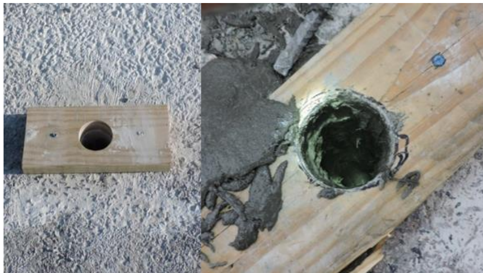
Figure 91. Pour holes for UHPC joints on the Wolf Creek bridge
