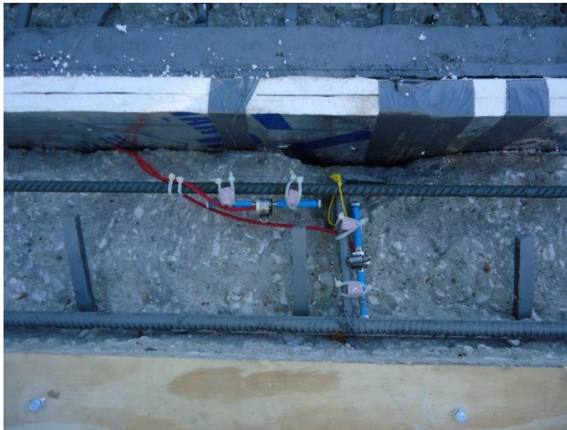
Figure 71. Strain gages within the joint header
