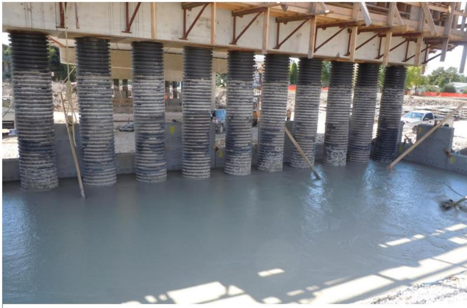
Figure 7. Backfill Construction with LDCC (from Loewen et al. 2012)
