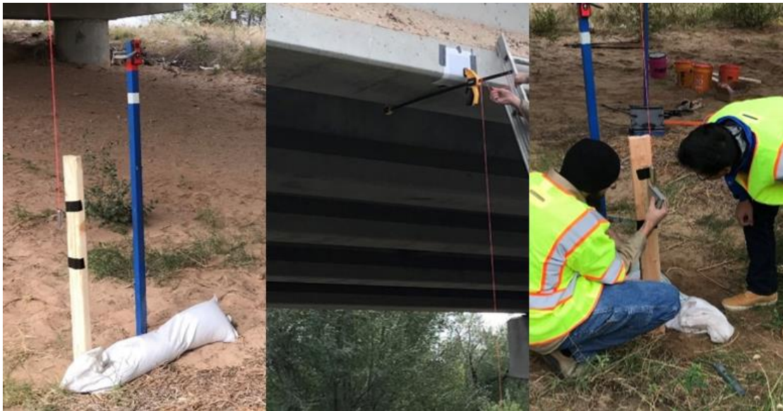
Figure 86. Laser measurer and plumb bob setup (left), clamp on the girder bottom (middle), and method used for measurement with the plumb bob (right)
