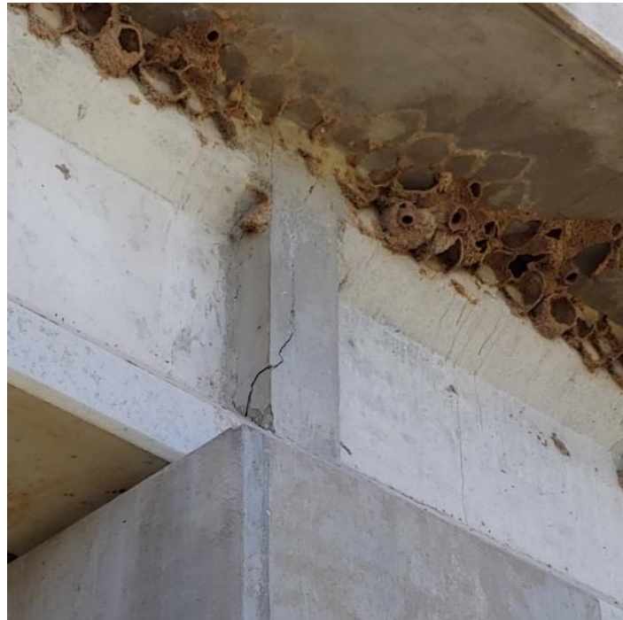
Figure 82. Example of positive moment cracking in a continuity joint of the U.S. 183/412 bridge over Wolf Creek
