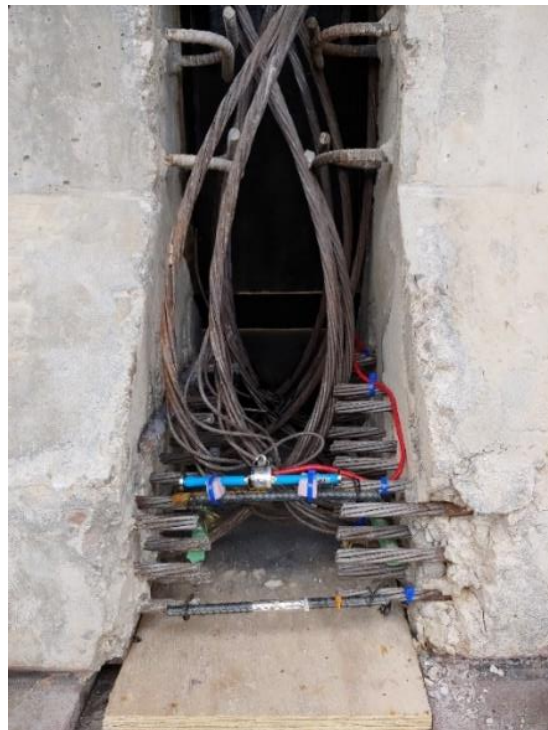
Figure 89. Strain gauge placement in the joint
