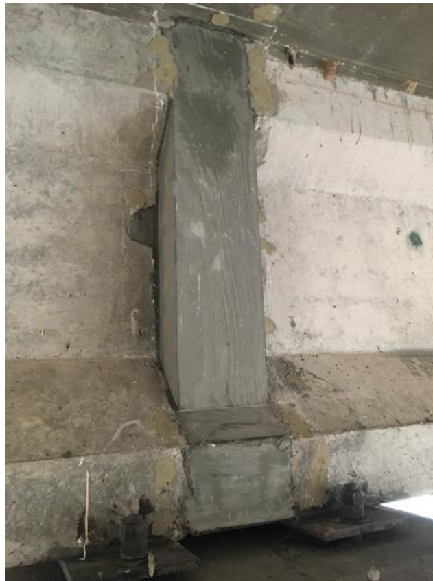
Figure 95. Completed UHPC continuity joint after form removal
