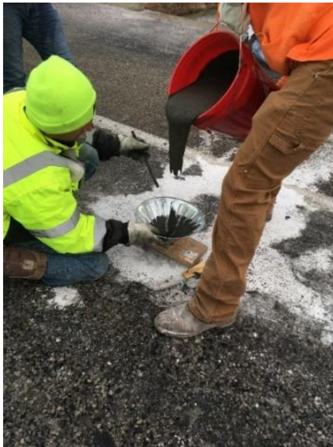
Figure 92. Placement of UHPC into fill hole in the bridge deck
