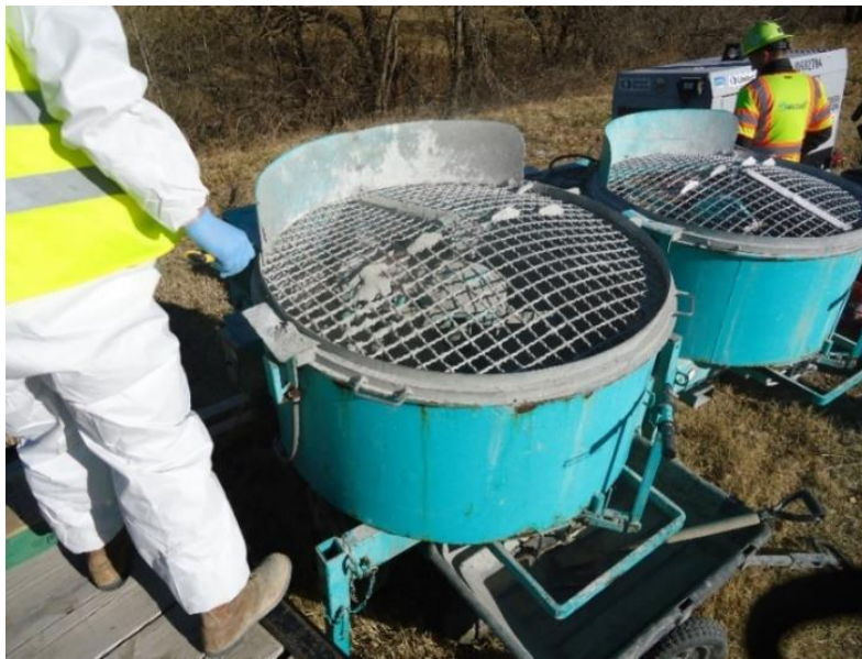
Figure 69. High shear mixers used for mixing UHPC
