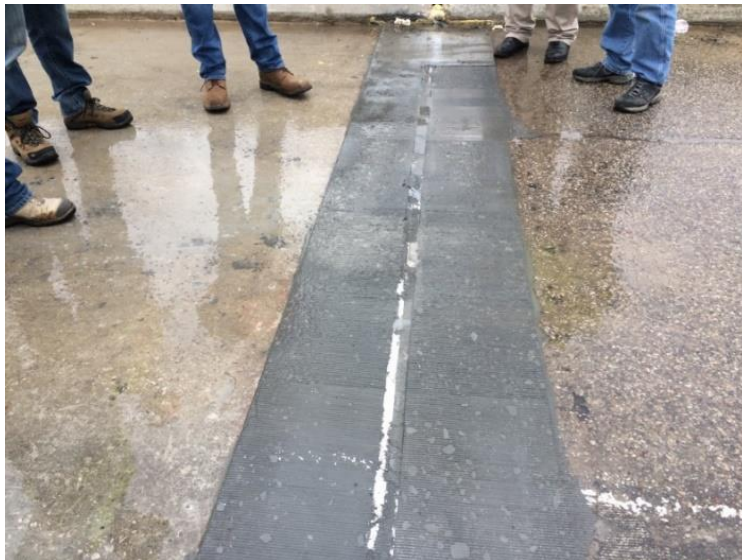
Figure 74. Entire Joint after grinding
