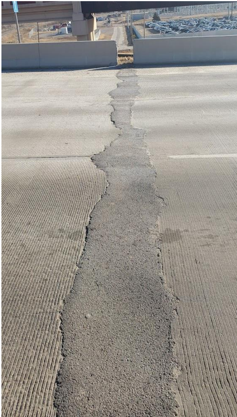
Figure 27. Shields Boulevard over I-40: Full depth asphalt pressure relief joint
