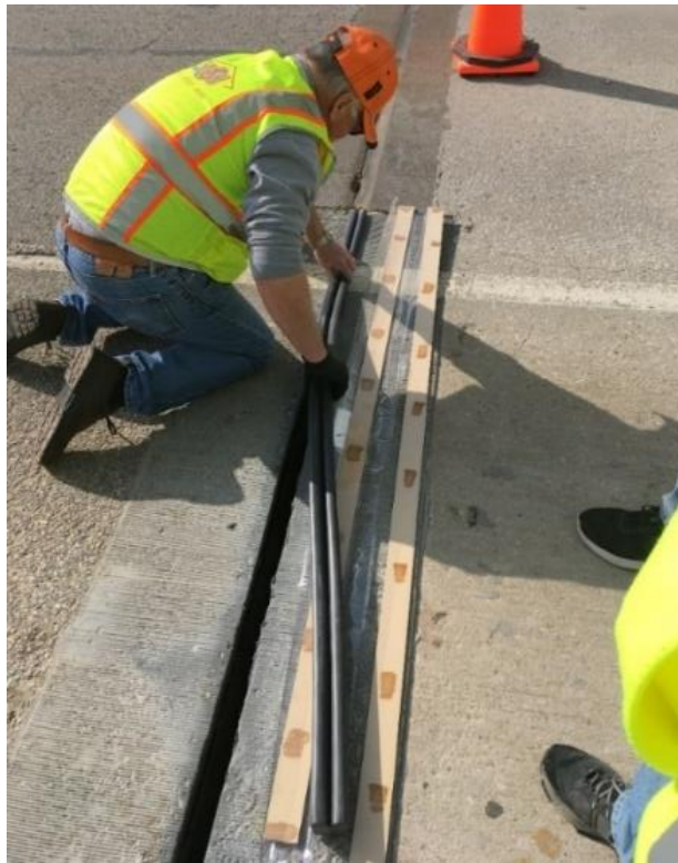
Figure 75. Installation of BEJS material by SSI Highway Products personnel
