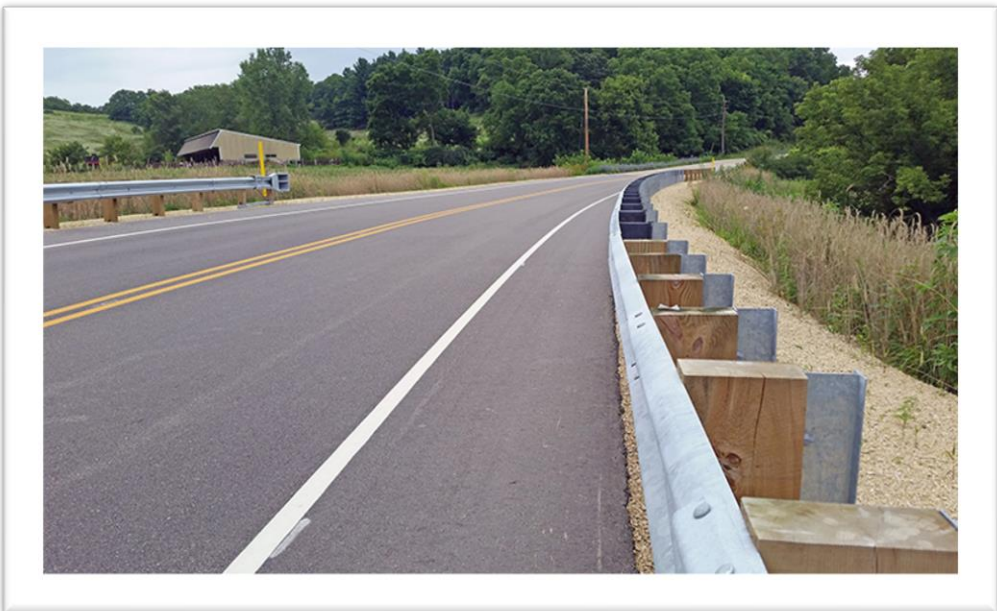
Figure 5.3. Rural Roadway with Barrier (Source: Ayres Associates, 2021)
