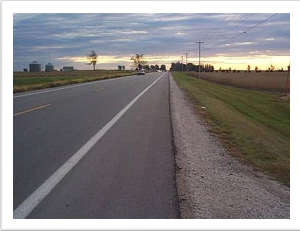
Figure 5.2. Rural Roadway with No Barrier (Source: FHWA, 2023)
