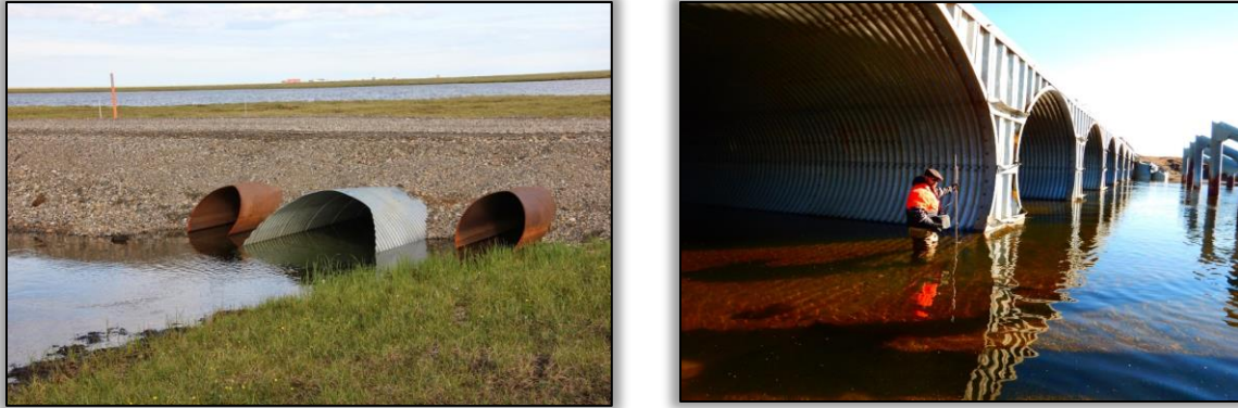
Figure 2.2 Photographs of culvert sites in Prudhoe Bay, Alaska
