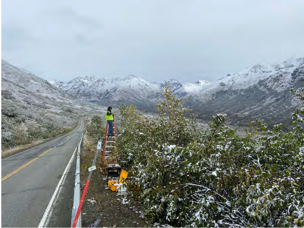
Hatcher Pass MP 15 station being installed. View looking northeast toward avalanche area.
