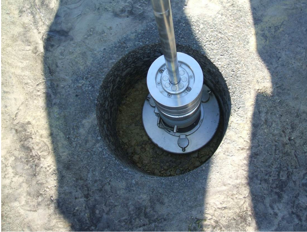
Figure 5. LWD testing on aggregate base through 16 in (406 mm) core hole.
