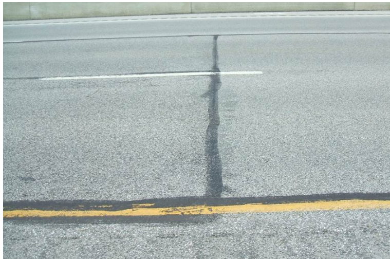
Figure 12. LAK-2 WB lane stabilized section looking north at construction joint.
