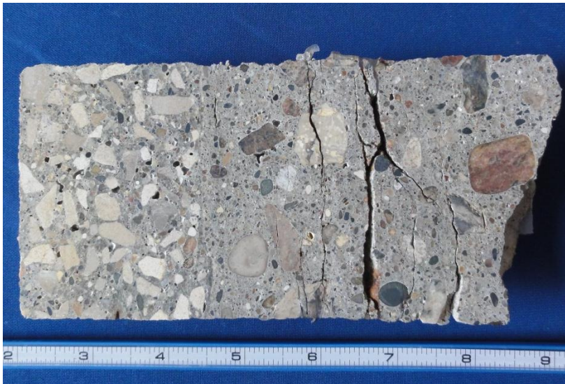
Figure 7. Lapped section of Core 42; top end is on the left of the photo. Numerous cracks due to corrosion and ASR are present in the base concrete; no cracking was detected in the topping concrete.
