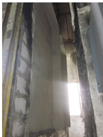
Figure 4. The 1 st test - exposed side
