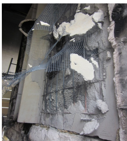
Figure 13. The 2 nd test - fire exposed side, after fire test
