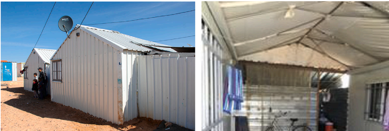
Fig. 1. T-shelter in Jordan [5].
