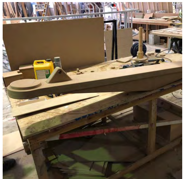
fig. 2.24 Fabricating seesaw from exterior grade MDF
