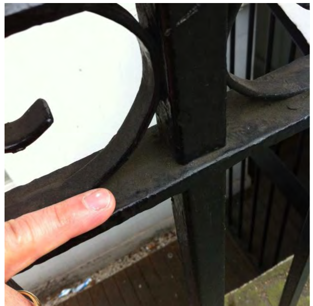
fig. 3.6 Using a finger to gauge scale
