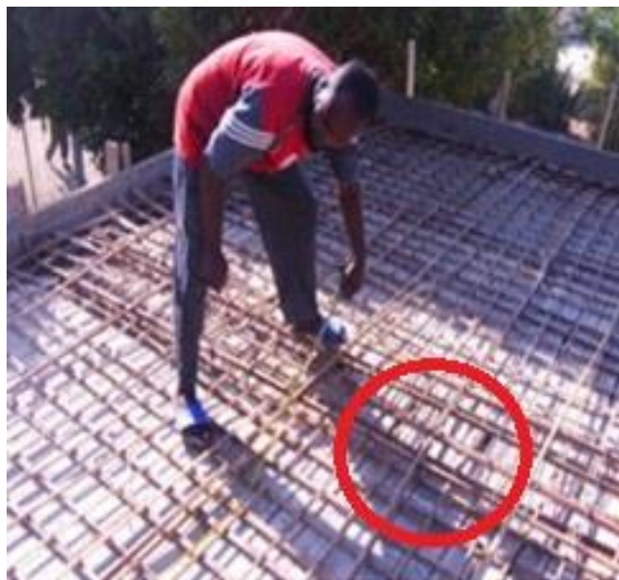
Figure 4.4 Intermediate beam Source: (Daoud, 2013)
