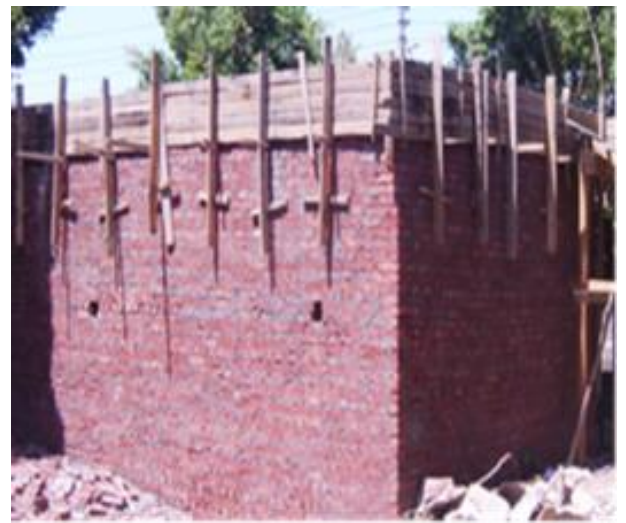
Figure 4.5 Final constructed building Source: (Daoud, 2013)
