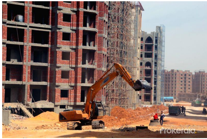
Figure 1.1 Construction of the New Administrative Capital
