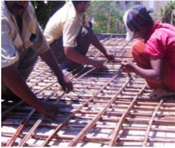
Figure 4.2 Slab reinforcement Source: (Daoud, 2013)
