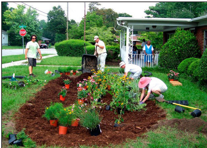
Figure 4.23: Rain garden being built in a residential front yard.
