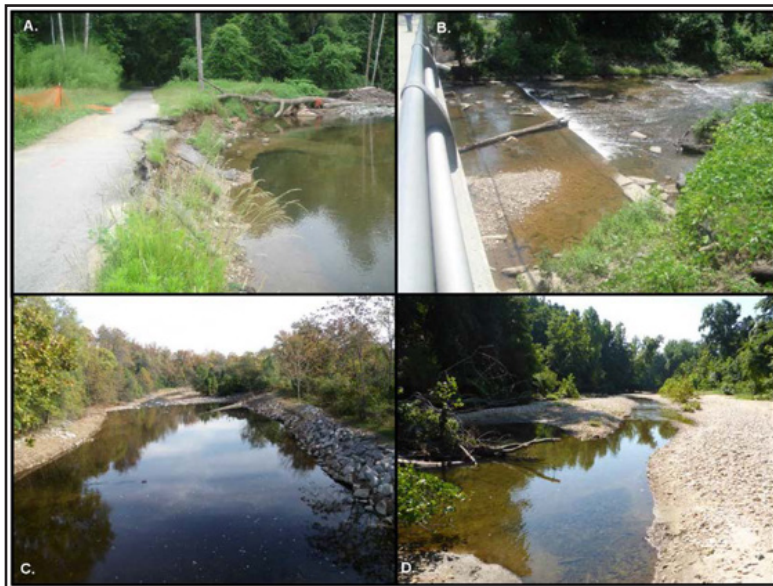
Figure 2.31: Portions of Anacostia tributaries impacted by Army Corps of Engineers channelization projects, showing erosion problems, fish blockages, and unhealthy aquatic habitats. Source: Army Corps of Engineers.
