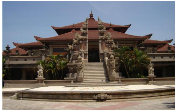
Figure 5. Ksirarnawa Building Condition
