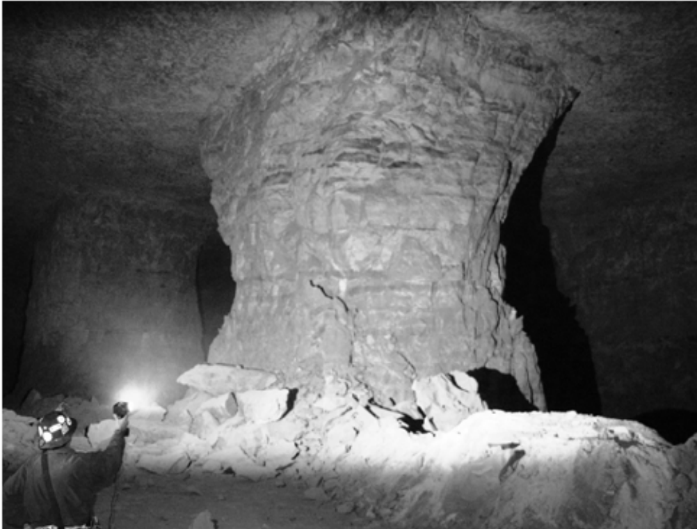
Figure 3.6: Photograph of a pillar with hourglass profile, a classical indicator of an overloaded pillar (from Esterhuizen et al., 2007).
