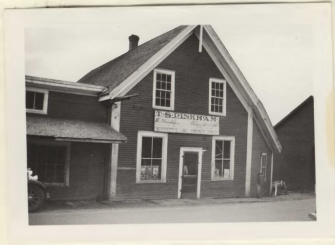
The general store of T.S. Pinkham and Company at Fort Kent Falls. This marks the site where the enterprising lumber busi- ness of Levi Sears and the subsequent owners was carried on. See page 31.
