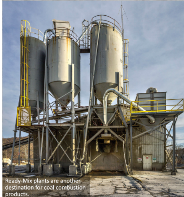
Figure 12. Concrete ready-mix plant.
