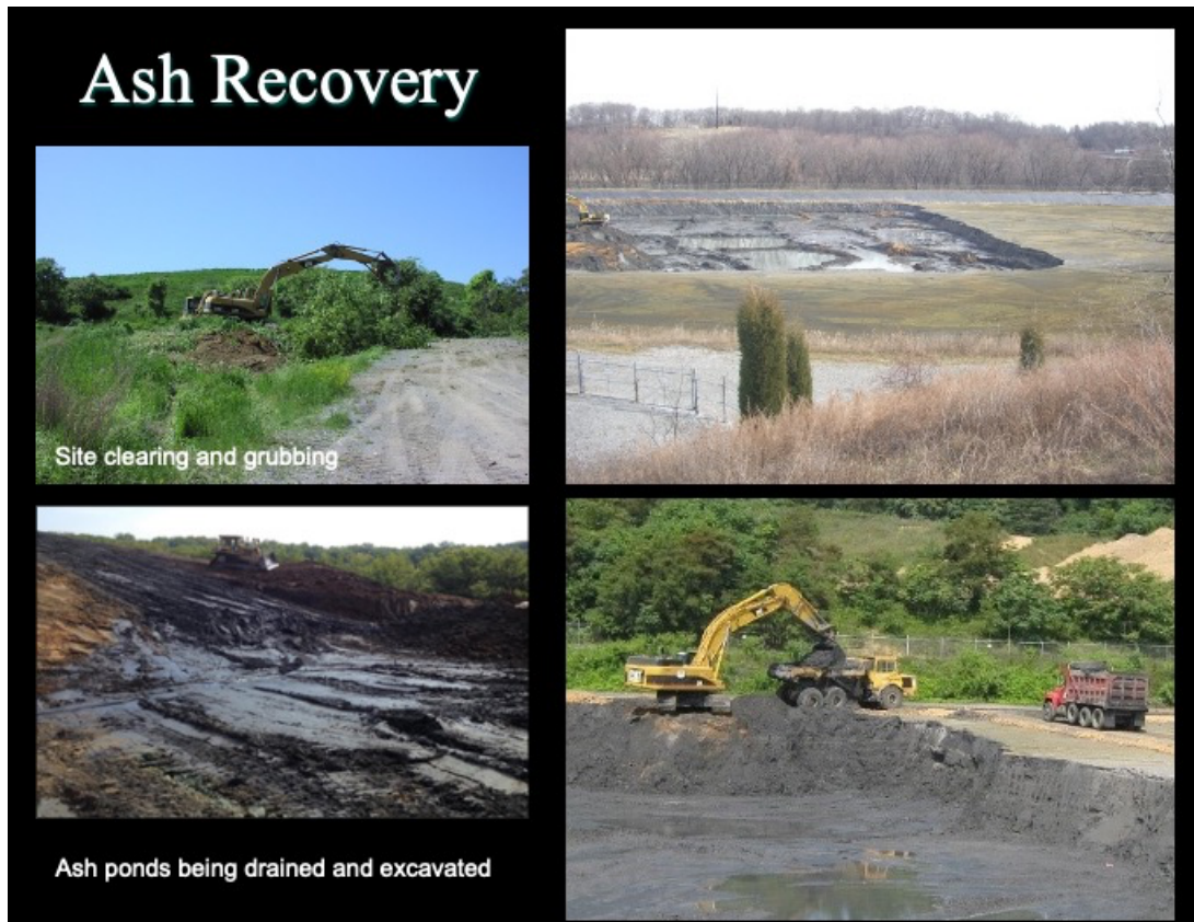
Figure 9. Views during ash recovery/harvesting at R. Paul Smith landfill.
