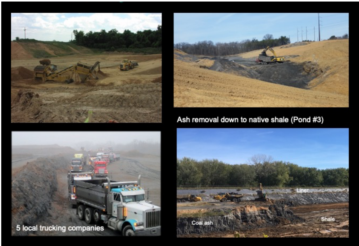
Figure 9 (contd). Views during ash recovery/harvesting at R. Paul Smith landfill.
