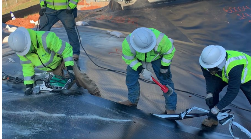
Figure 3: Geomembrane seaming in progress – tape removal (right) ahead of seaming (left).
