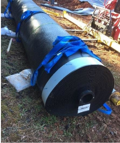
Figure 2: Geomembrane with taped edge.
