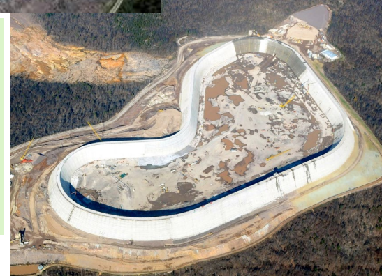
Taum Sauk During Repair - Cement, Fly Ash & RCC
