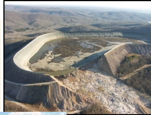
Taum Sauk During Repair - Cement, Fly Ash & RCC
