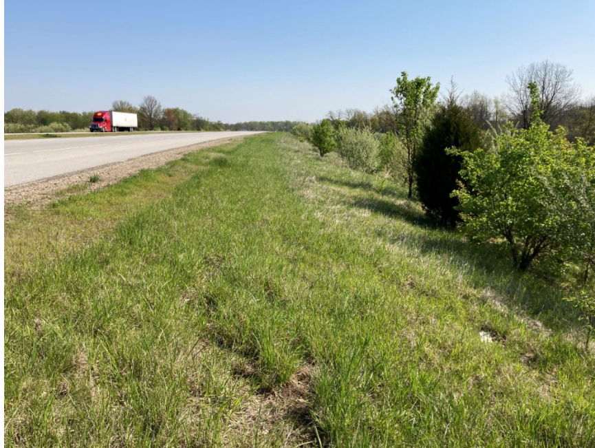
Figure 9. Post Construction Performance of Fly Ash Embankment
