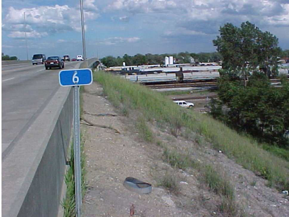
Figure 3. US12/20 Bottom Ash Embankment in Lake County (Picture taken in 2002).
