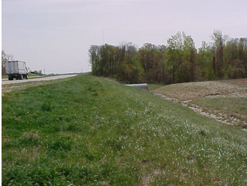
Figure 8. Post Construction Performance of Coal Ash Embankment
