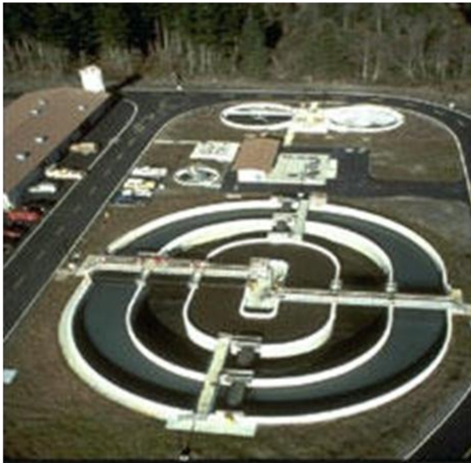
Figure B49. Enhanced Nutrient Removal Treatment Technology.
