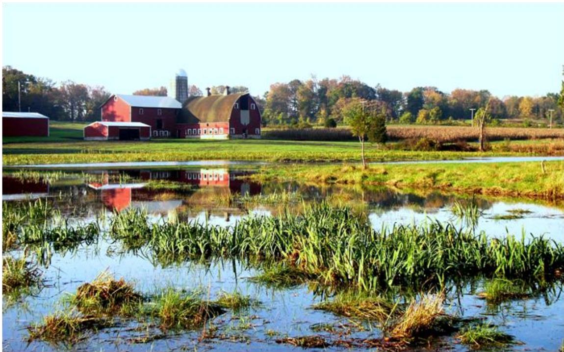
Figure B23. Constructed wetland.
