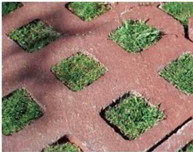
Figure B38. Permeable pavements.
