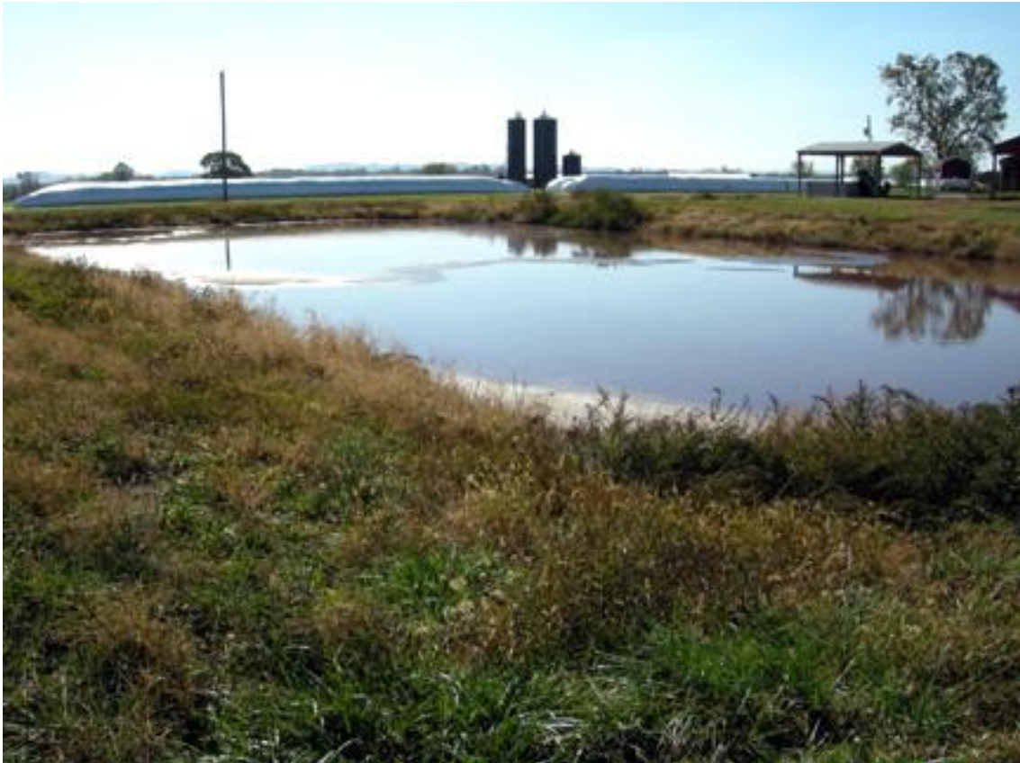
Figure B22. Waste treatment lagoon.
