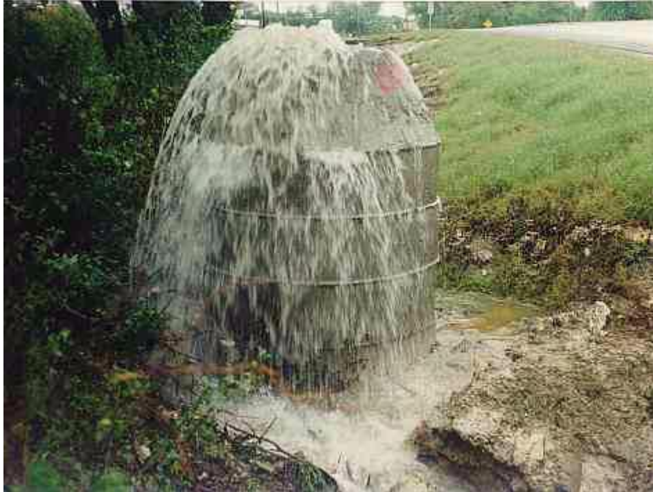
Figure B45. Sanitary Sewer Overflow.
