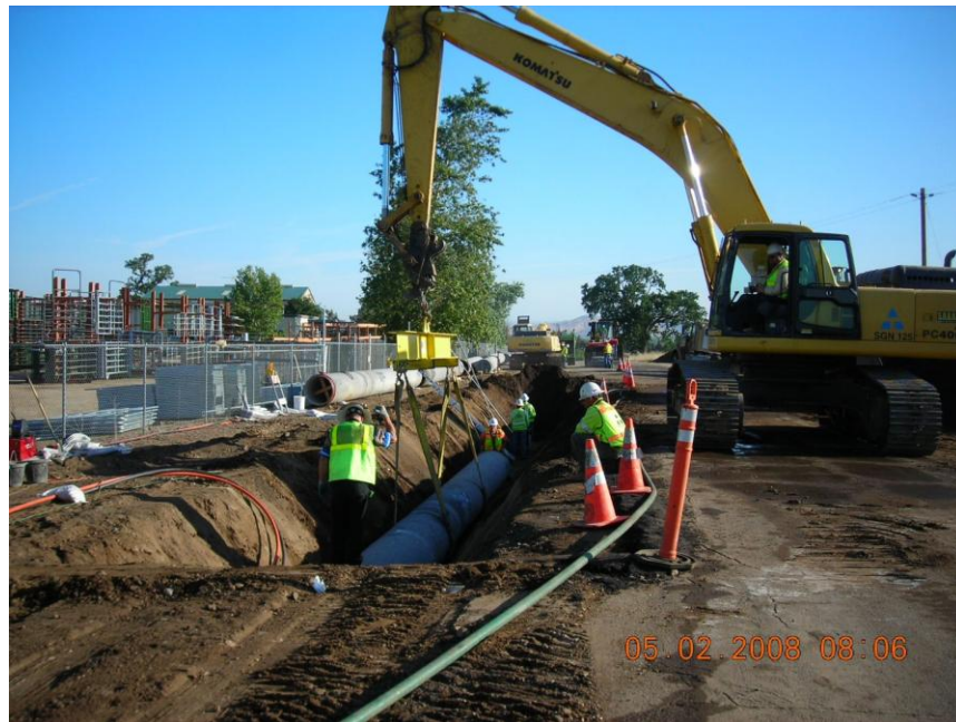
Figure B47. Sewage pipe being replaced.
