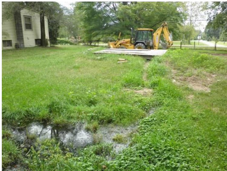
Figure B44. Failing septic system.
