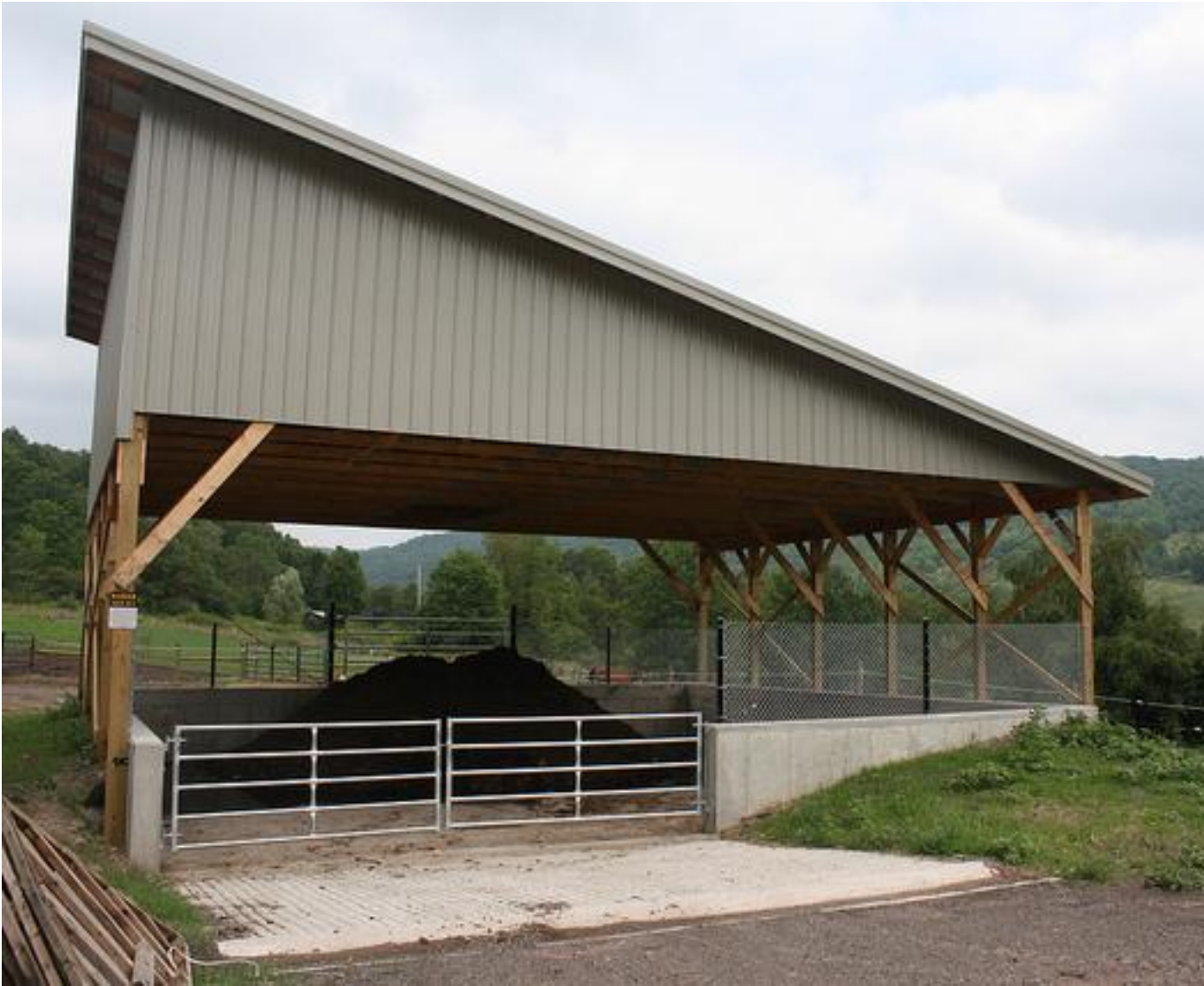
Figure B14. Manure storage facility
