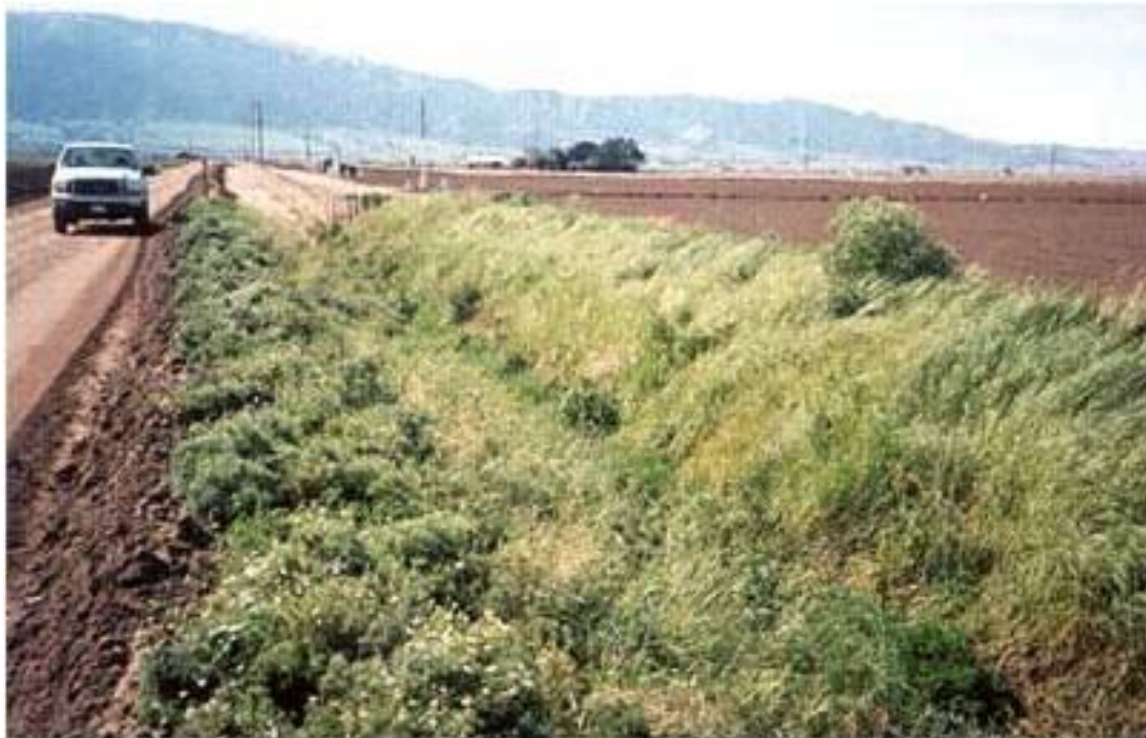
Figure B21. Grassed waterways.
