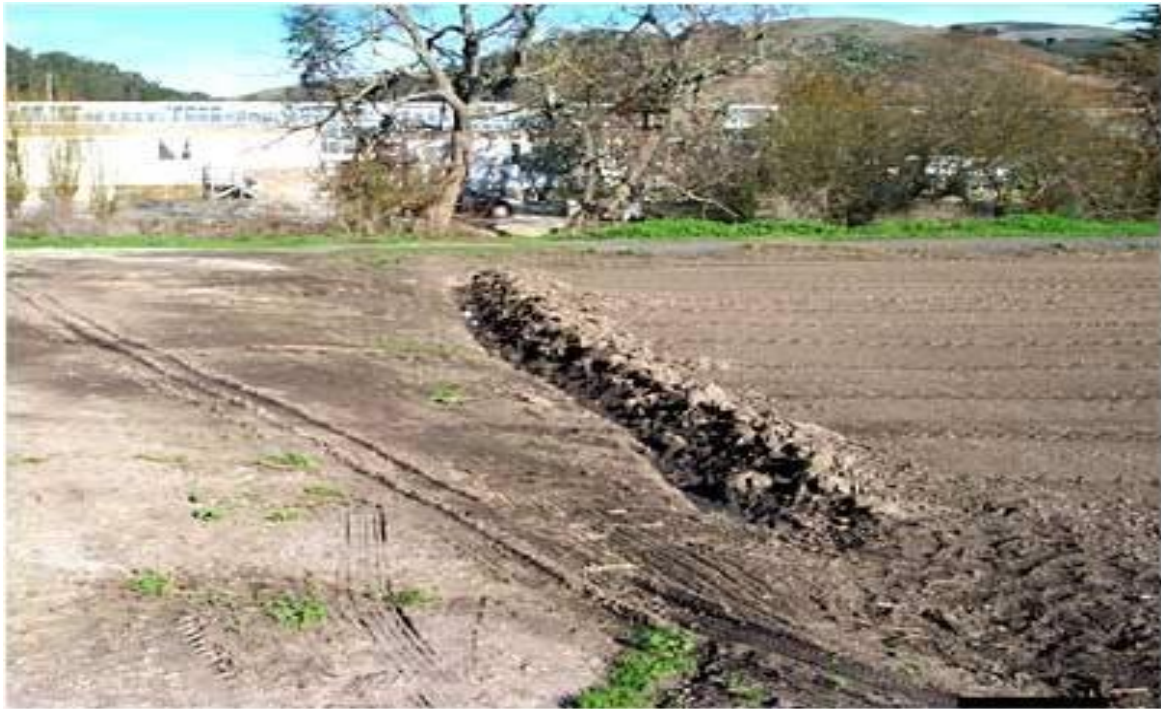
Figure B20. Earthen diversion
