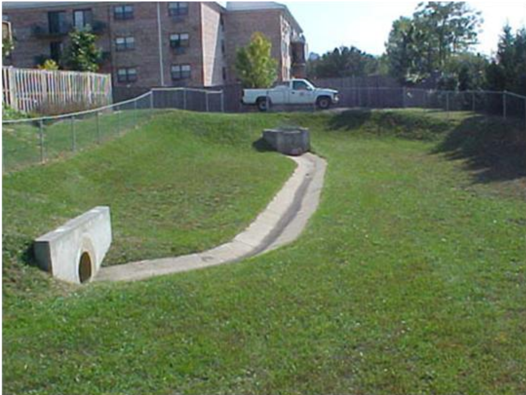
Figure B43. Dry detention basin designed to temporarily detain runoff during storm events.
