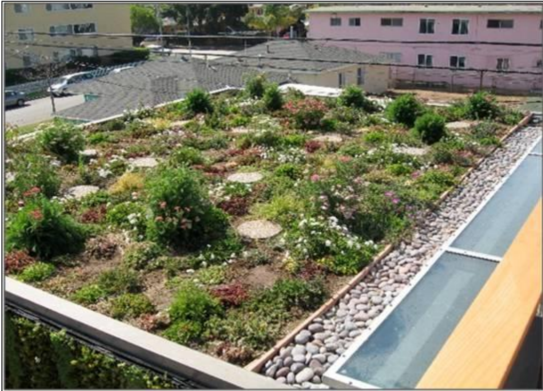
Figure B39. Green roof in urban area.
