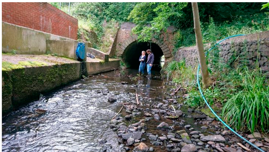
FIGURE 3 The monitoring location on the Bourn Brook during summer low-flow conditions.
