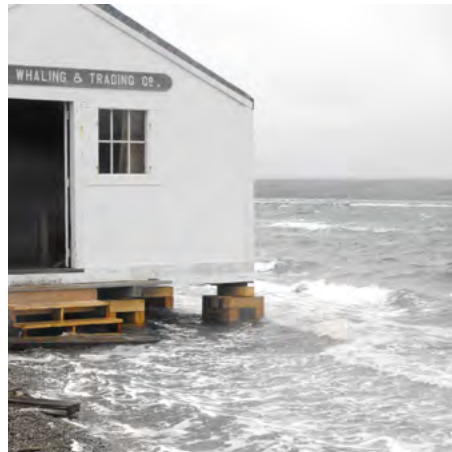
2016 during storm, high water level. This has never been witnessed in the history of the park.
