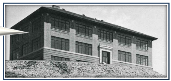
Metallurgy Building had classrooms, laboratories for metallurgy, ore dressing and chemistry in 1923-1987
