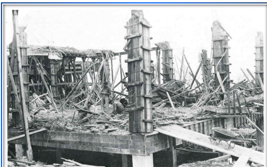
Wreckage of Metallurgy Building floor slab collapse, 1920.
