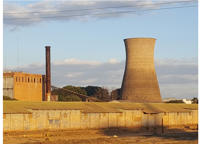
A coal fired plant in Lusaka. The Zambian government has sought to diversify its electricity generation sources away from complete reliance on hydroelectric power. Coal accounts for 11% of electricity power generation today.
