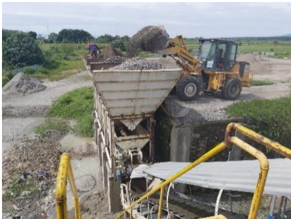
Dumping material ke aggregate bin di batching plant
