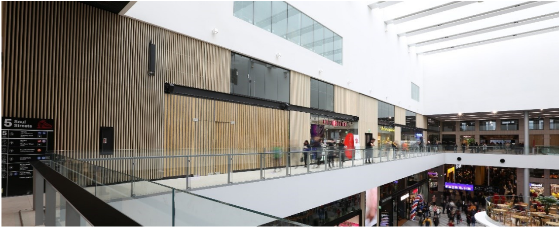
Figure 9 Pasila station in Helsinki (Puucomp, 2022)
