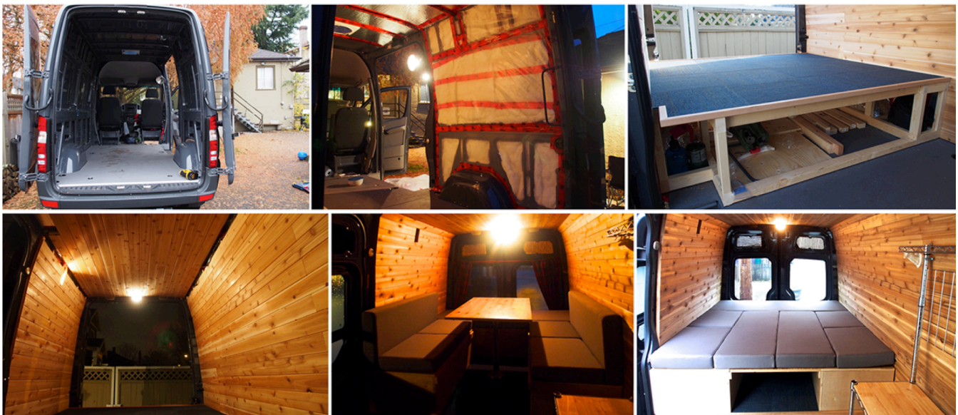
Figure 1. Building steps: From top left: the empty van; step 1 – wall insulation; step 2 – back storage platform; step 3 – wall finishing with cedar panels; step 4: benches-table-bed unit in a) table position, b) bed position.
