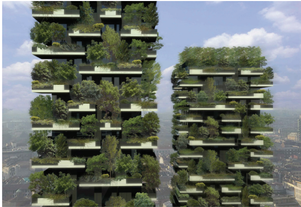
Fig. 7. Bosco Verticale (Vertical Forest) by Boeri Studio (Stefano Boeri, Gianandrea Barreca, Giovanni La Varra). 21
