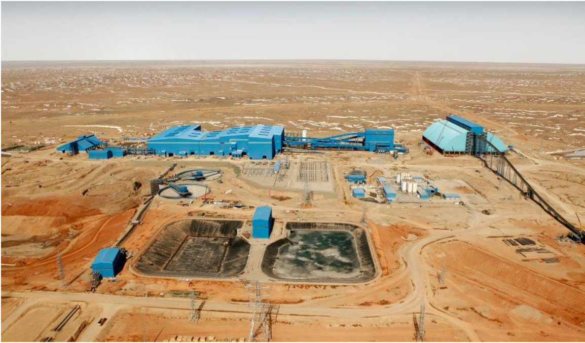
Figure 3.7. OT extraction facility along with liquid mine waste storage ponds.
