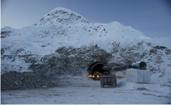
Figure 6 West Portal Dvoynoye Mine
