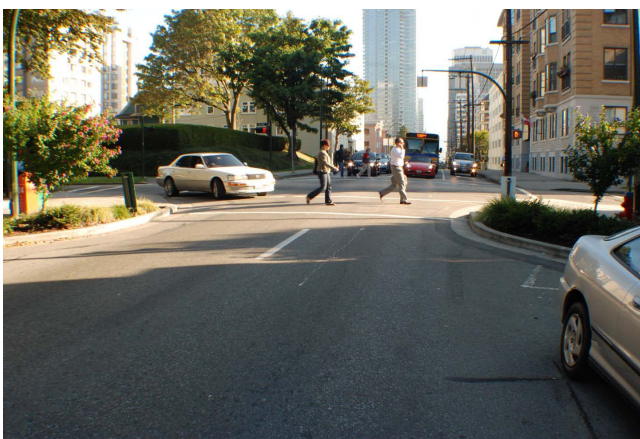
Figure 3 A location with a corner bulge in place.
