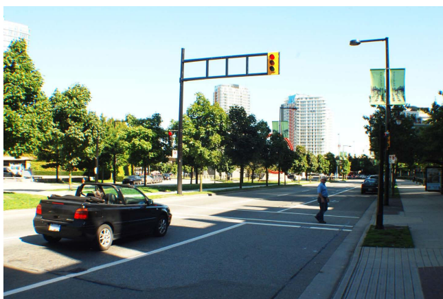
Figure 5 A signalized crosswalk and median at a midblock location on Expo/Pacific Blvd.
