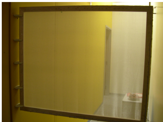
Figure 26: The fabric screen installed in a hallway. Each side of the screen is laced with conductive fabric.
