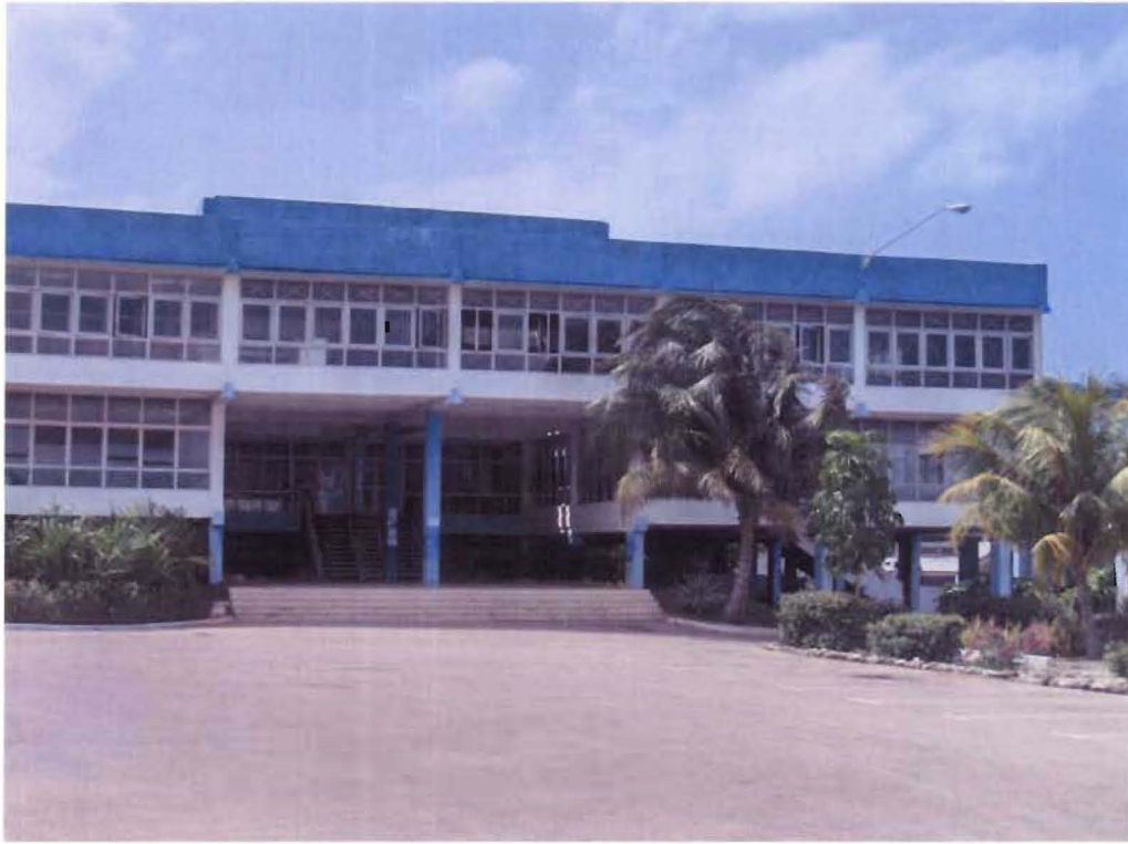
(Fig. 11) Main Entrance to ELAM.
