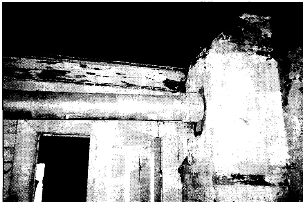
NE12 Neubergthal. Southwest corner of room A2 with chimney structure, heating pipe, and door to A1.
