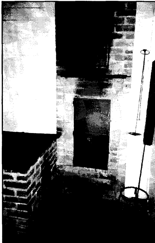
Teichroeb House. Brick heating oven (A6).
