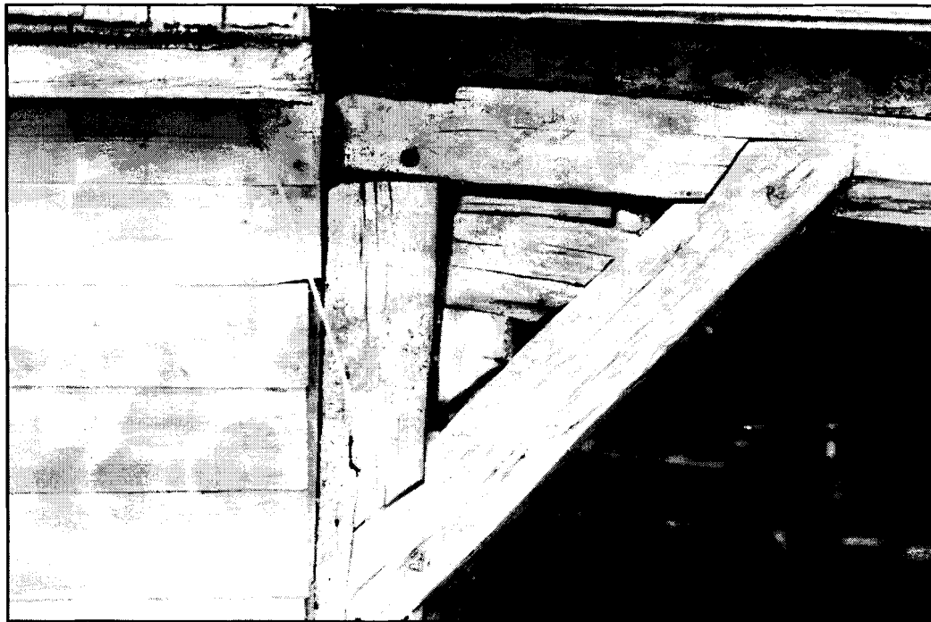
70 Chortitz Rd. South. Diagonal brace, South side of dwelling.
