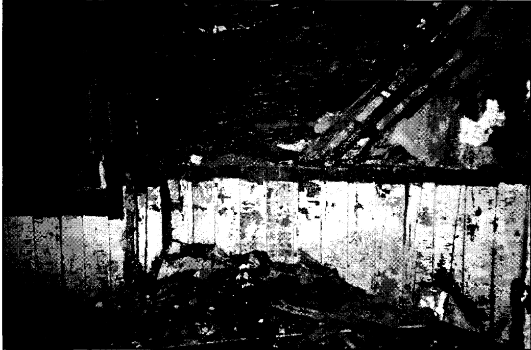
70 Chortitz Rd. South. Wainscoting and wall construction, North wall of A1.
