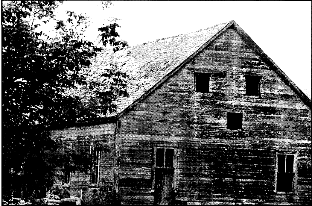
60 Chortitz Rd. South. East end of dwelling.
