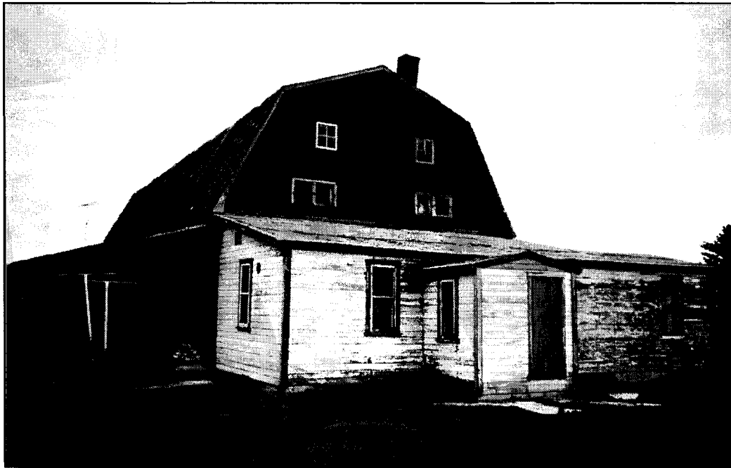
NE14 Neuberghal. South end of housebarn. White lean-to is dwelling section. The two horizontal windows in barn just above the dwelling are second floor of dwelling (B1 and B2).
