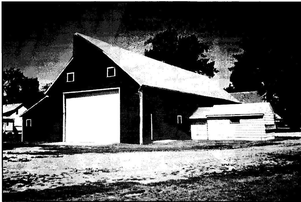
164 Reinland Ave. Southeast corner of housebarn.
