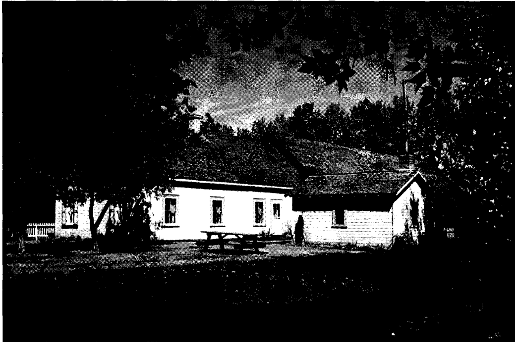
Teichroeb House. Dwelling and Summer Kitchen.
