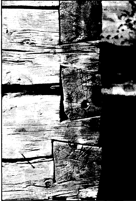
26 Chortitz Rd. South. Dove tail joints, Southeast corner of dwelling.
