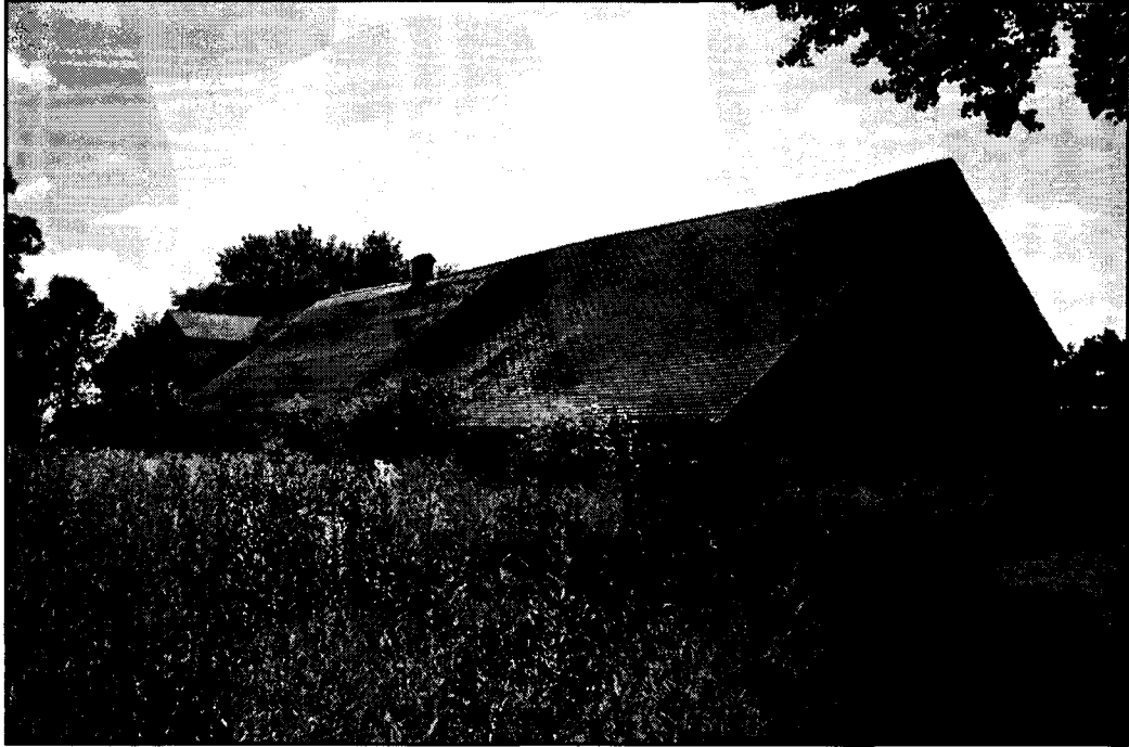
SW3 Neuberghal. Northwest corner of housebarn (barn section).
