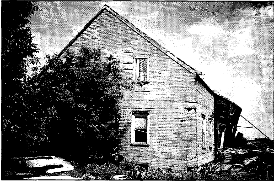
Driedger Housebarn. West end of dwelling.
