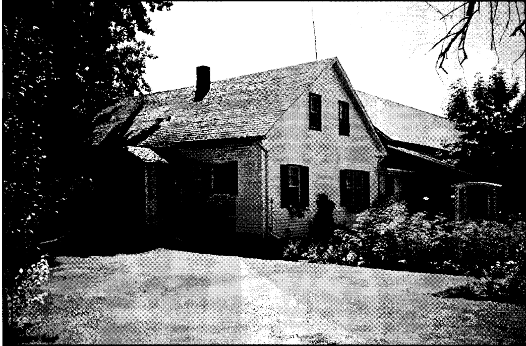
164 Reinland Ave. The dwelling facing the street in this “T-shaped” housebarn exhibits a front door, vestibule and asymmetrical facade.
