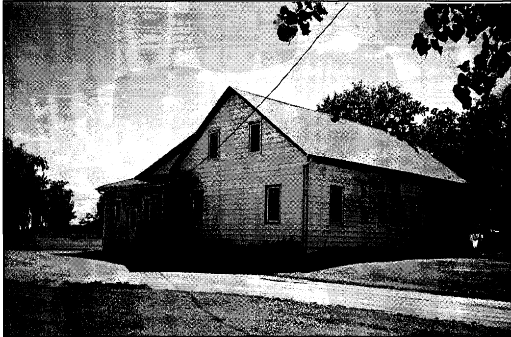
170 Reinland Avenue. Northeast corner of dwelling.
