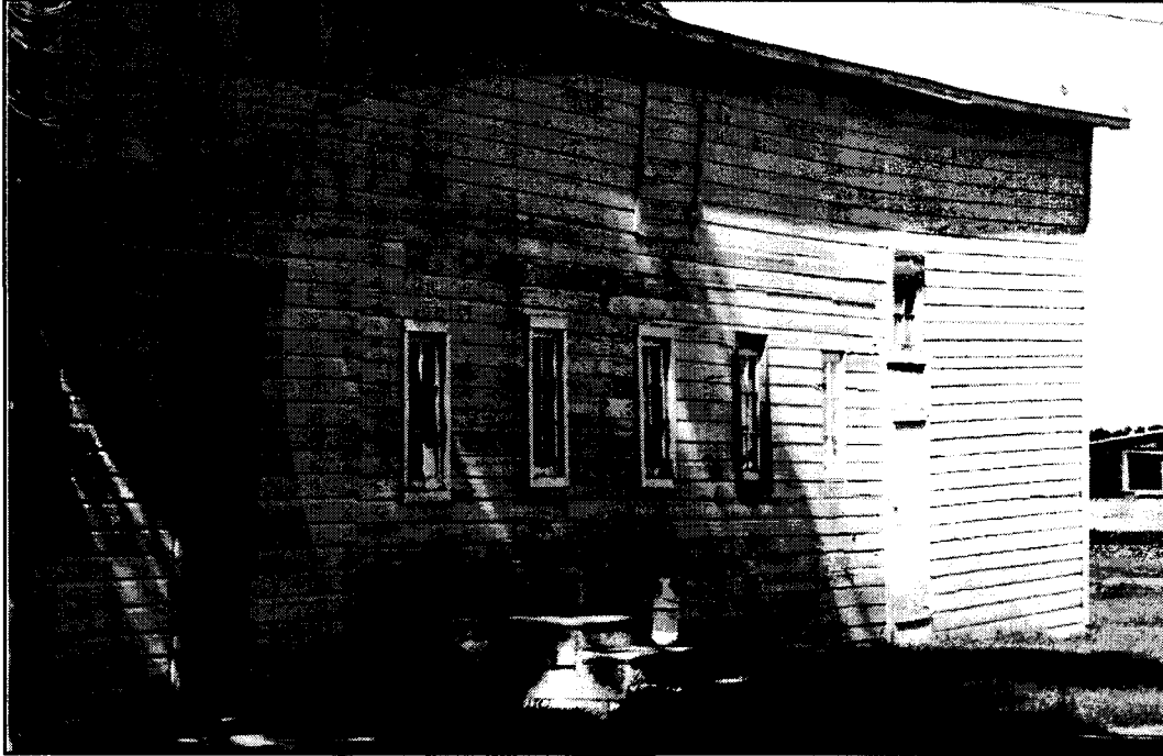
NE12 Neuberghal. South side of housebarn. Door on left side is entrance to A1.
