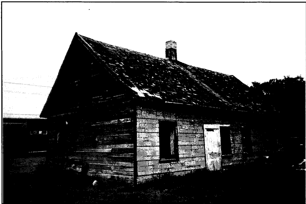
SW4 Neuberghal. Southwest corner of dwelling.
