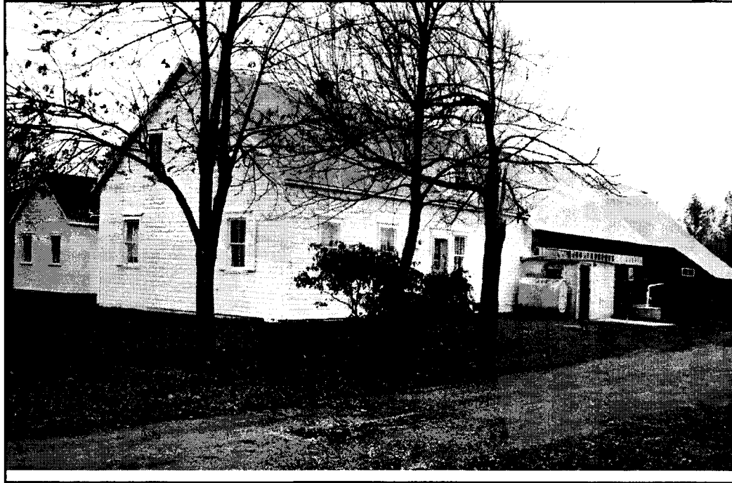
141 Reinland Ave., Southeast corner of housebarn
