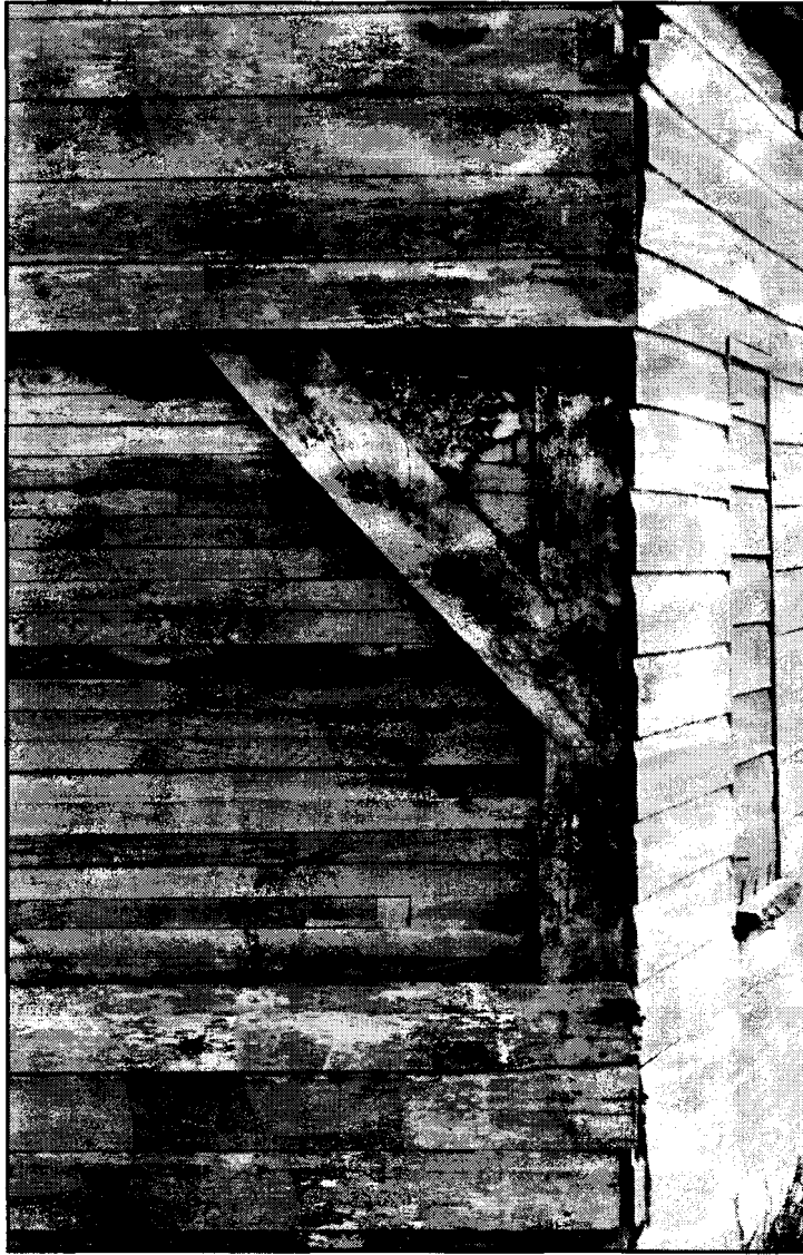
NE3 Neubergthal. Exposed crib wall construction with diagonal brace beams, northwest corner.
