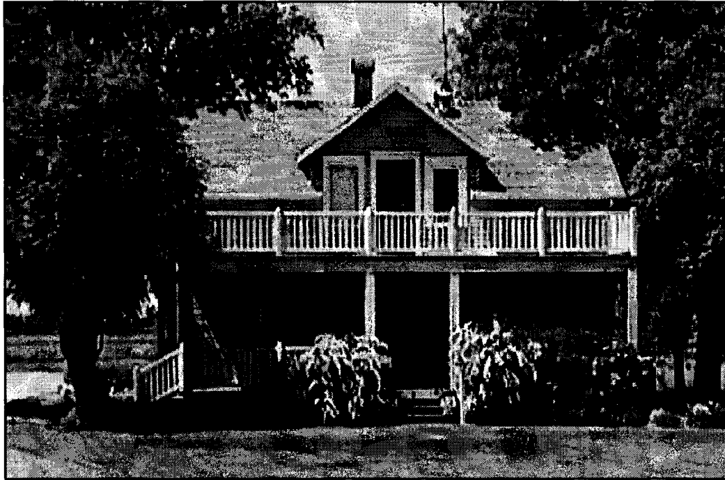
NW4 Neubergthal. East side of dwelling of housebarn. Symmetrical facade with front door of this "T-shaped" housebarn face the street.
