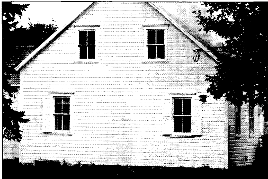
141 Reinland Ave., South facade of housebarn. The lack of a door and the symmetry of the end of the dwelling facing the street displays a modest, formal and closed facade.
