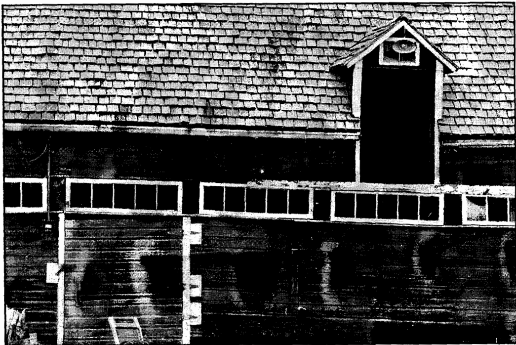
SE3 Neuberghthal. South side of barn.
