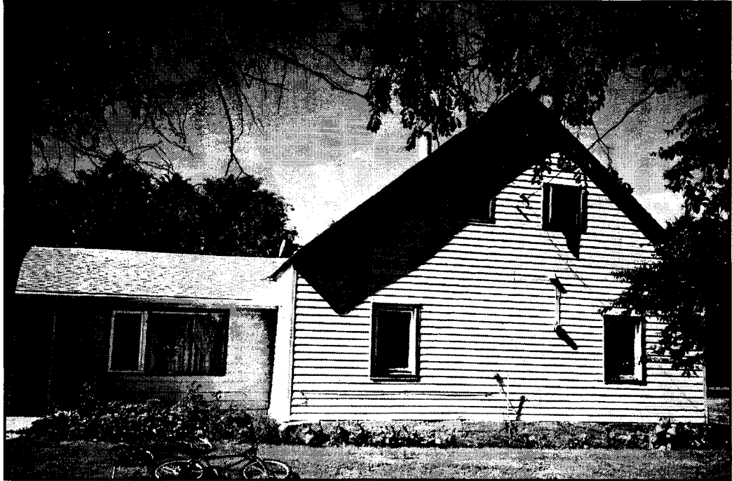
52 Chortitz Rd. North. East end of dwelling.
