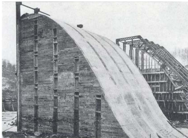
The Dam’s structure, designed to facilitate the flow of water.
