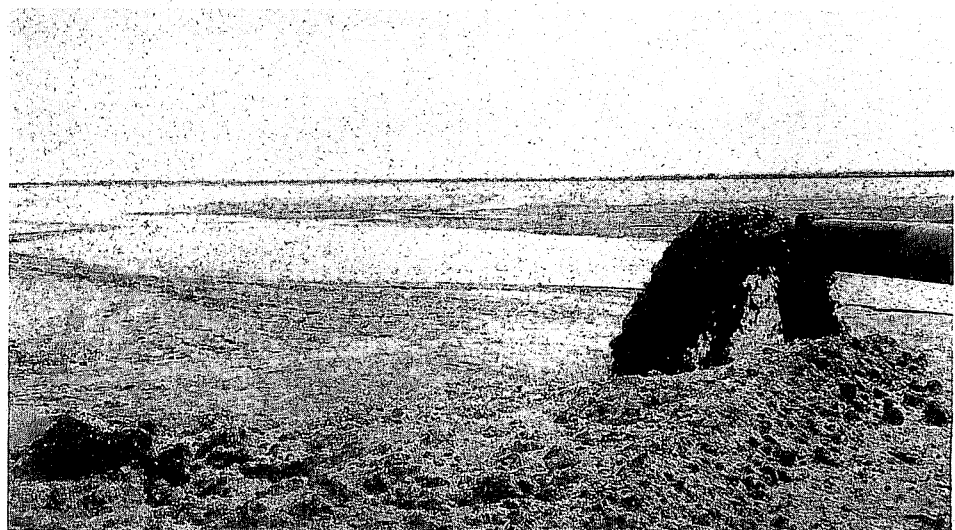
Dredged material from Baltimore Harbor gushes into the expansive North cell of Hart-Miller Island.
