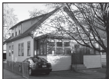
KILLARNEY 93 Pinehurst Avenue
