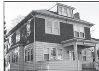
TOLLAMORE 138-140 Radcliffe Avenue
