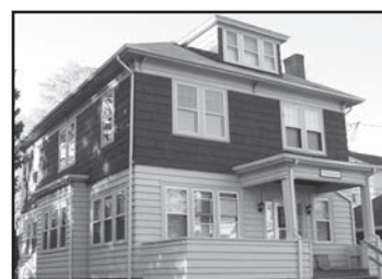
TOLLAMORE 138-140 Radcliffe Avenue
