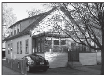
KILLARNEY 93 Pinehurst Avenue
