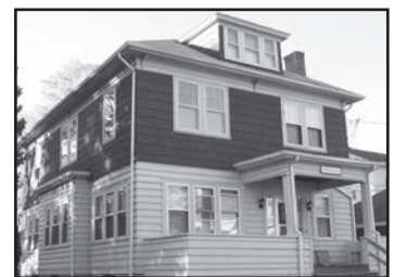
TOLLAMORE 138-140 Radcliffe Avenue
