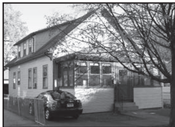
KILLARNEY 93 Pinehurst Avenue
