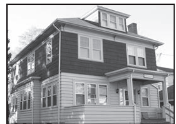
TOLLAMORE 138-140 Radcliffe Avenue
