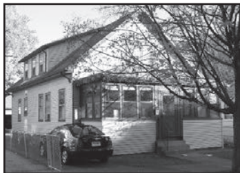
KILLARNEY 93 Pinehurst Avenue
