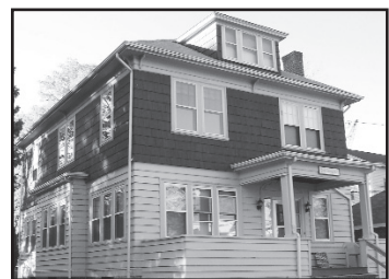
TOLLAMORE 138-140 Radcliffe Avenue
