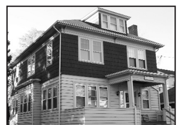
TOLLAMORE 138-140 Radcliffe Avenue
