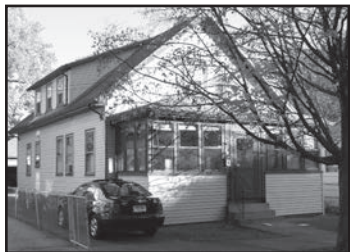
KILLARNEY 93 Pinehurst Avenue
