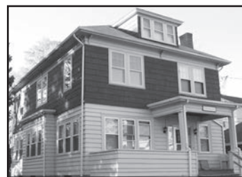
TOLLAMORE 138-140 Radcliffe Avenue
