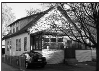
KILLARNEY 93 Pinehurst Avenue
