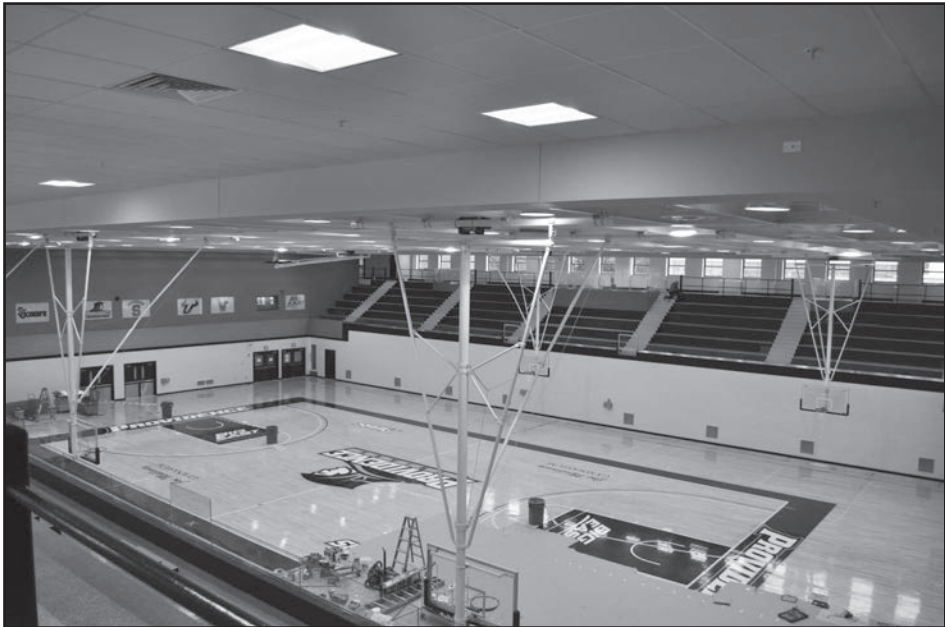
Renovations are nearly complete on the Mullaney Gymnasium in Alumni Hall.
