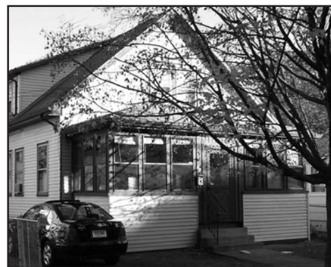
KILLARNEY 93 Pinehurst Avenue
