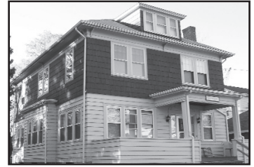
TOLLAMORE 138-140 Radcliffe Avenue
