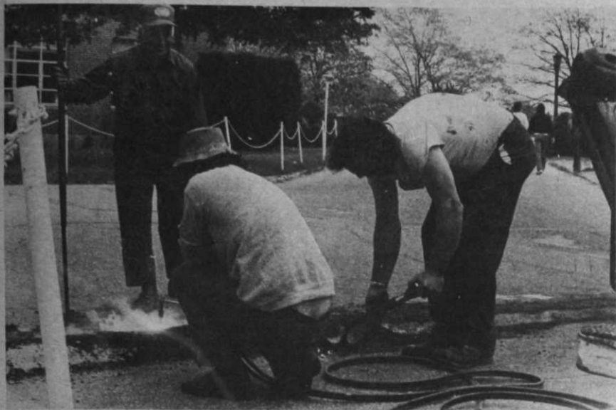
"Take a little more off the top, Joe!" Workers repair one of the traffic control bumps on campus last week.
