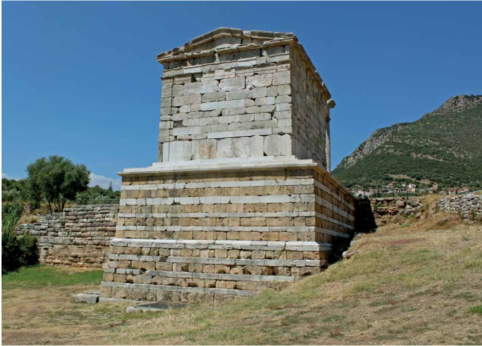
Figure 2. The restored podium of the heroon and the Messenian city wall (photo author).
