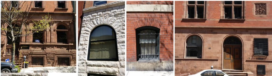
Figure 52 A small sampling of the variety of brick and stone archways found on one side of the street in one city block in Mt. Vernon Baltimore. Baltimore is known as a brick town. Images by Rebecca Habtour
