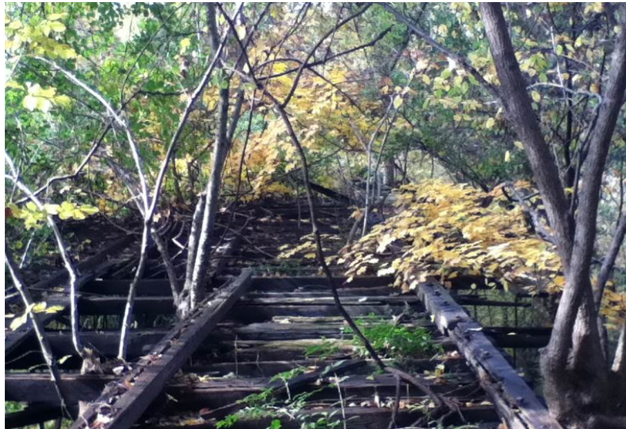
Figure 53: Nature Reclaiming Trestle Bridge Image by Author
