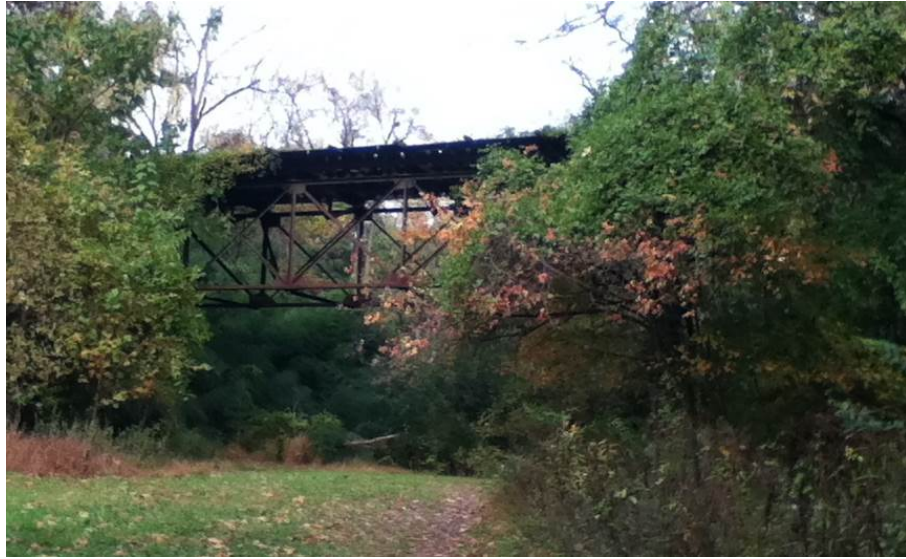
Figure 52: Trestle Bridge Entry to Glover-Archbold Park Image by Author
