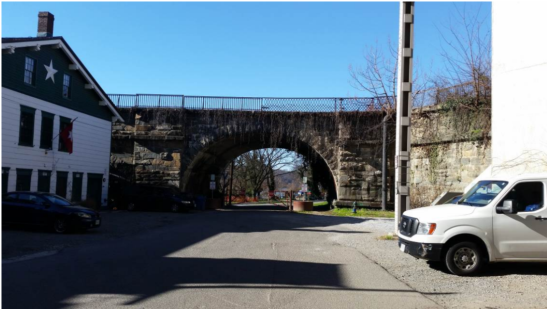
Figure 64: Aqueduct Abutment Image by Author
