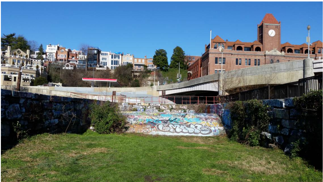
Figure 68: Abutment View to Georgetown Image by Author
