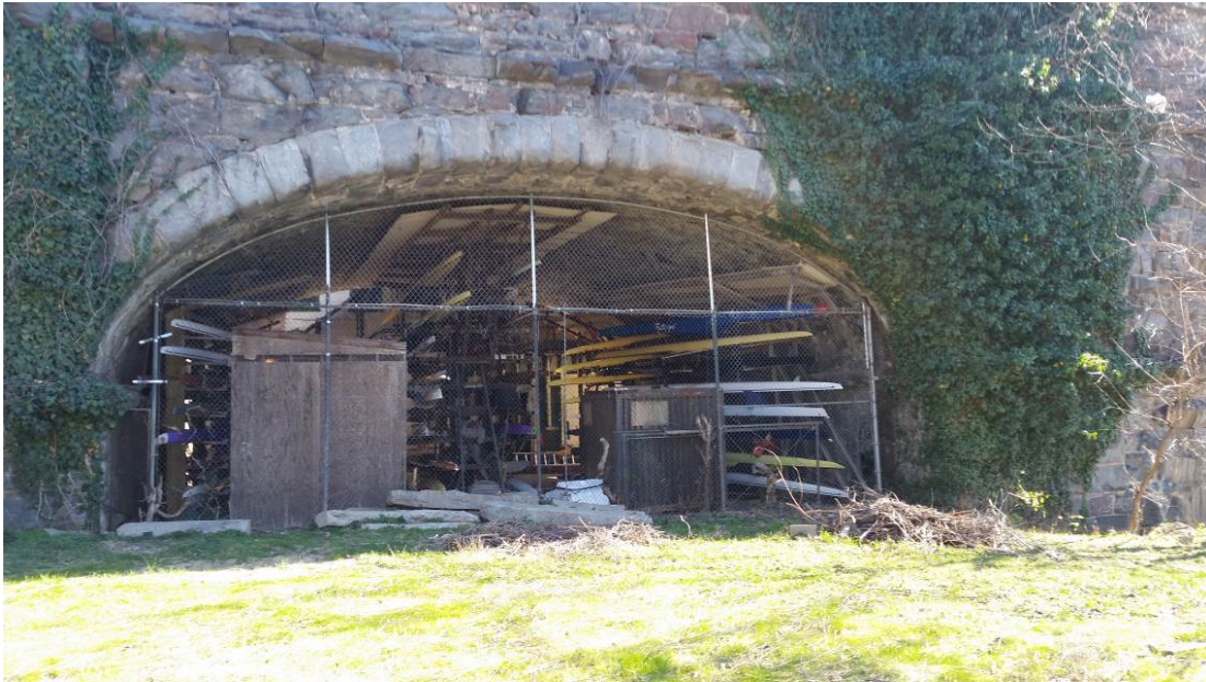
Figure 66: Aqueduct Abutment as Storage Image by Author
