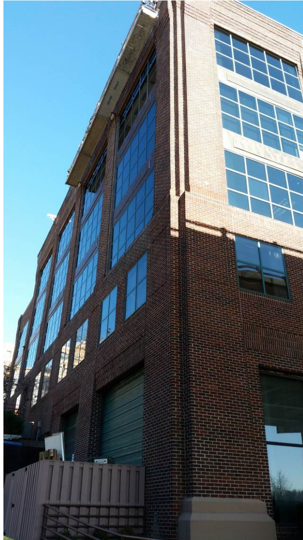
Figure 70: Industrial Character Along Water Street Image by Author
