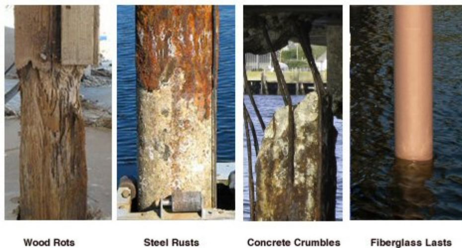
Figure 3 – Corrosion resistance of the FRP piles compared to other materials (Pearson Pilings 2016)
