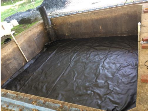
Figure 3.2. Placement of geotextile on top of the 1.2 m crushed stone
