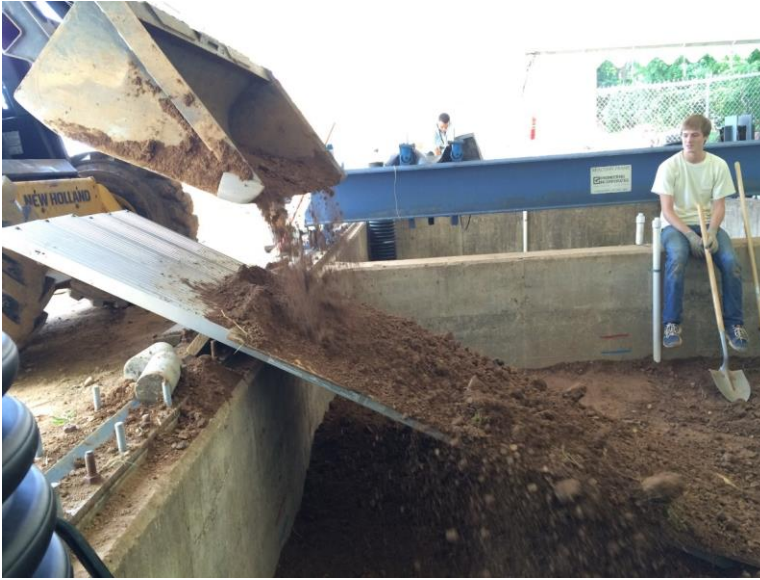
Figure 3.10. Use of ramp for transferring the material into the pits
