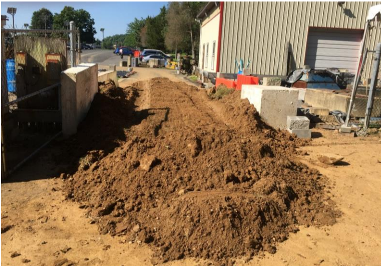
Figure 3.5. Spreading the ALF stockpile for drying prior to compaction
