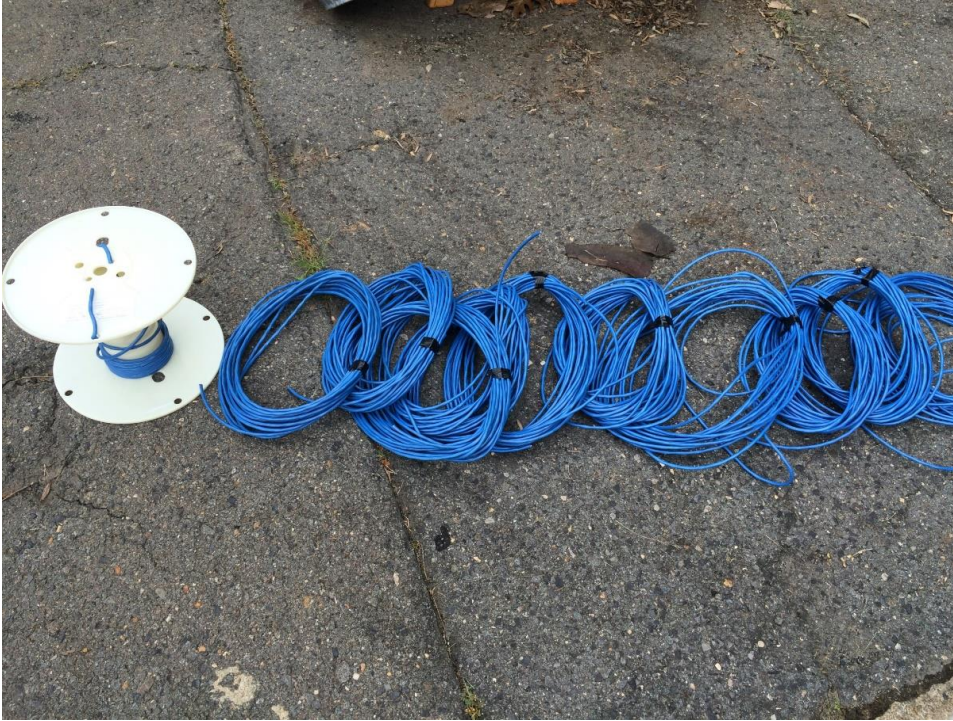
Figure 2.63. Thermocouple wires cut to length
