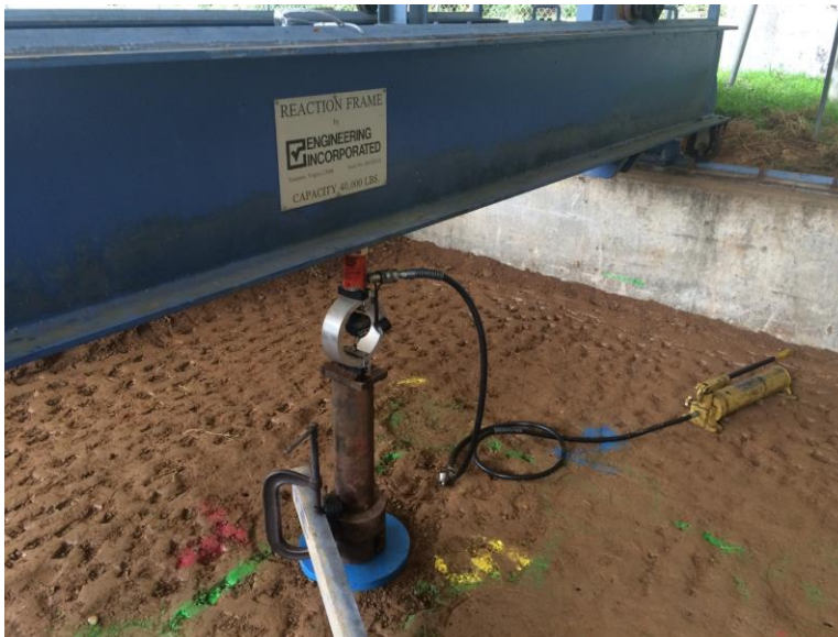
Figure 4.17. Static plate load test
