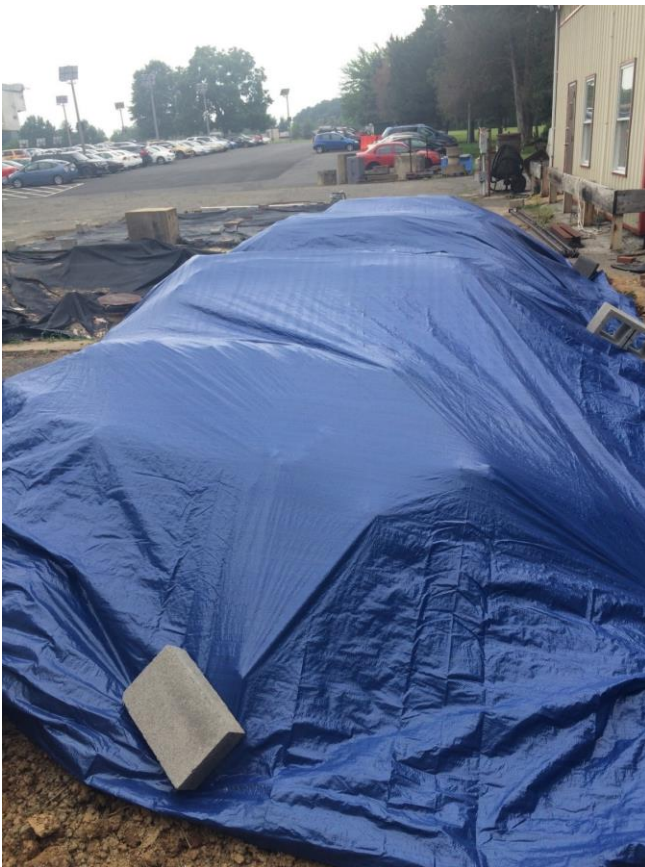
Figure 3.9. Covering the stockpiles
