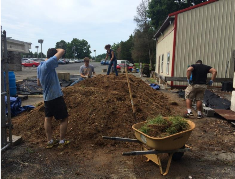
Figure 3.4. ALF stockpile--removing the organic soil from ALF soil
