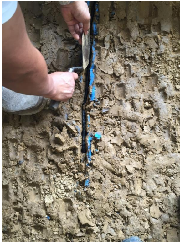
Figure 4.12. Cutting the HPC soil for embedding the thermocouple sensor
